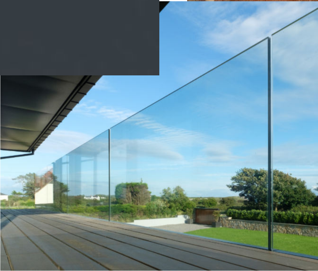
Frameless glass balustrading to veranda and balconies
