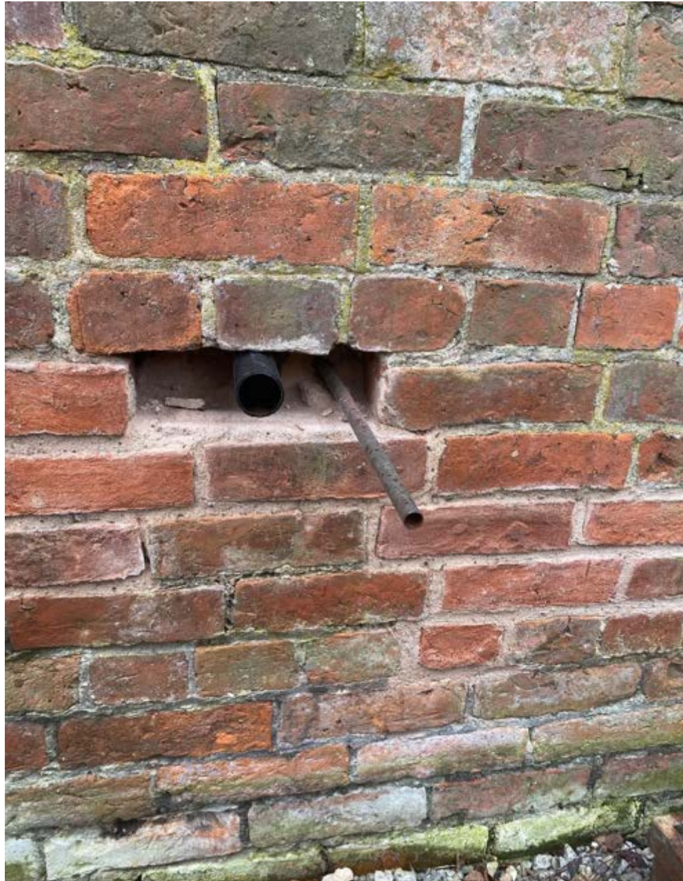
Figure 25 – Closer view of the removed brick and installed piping.
