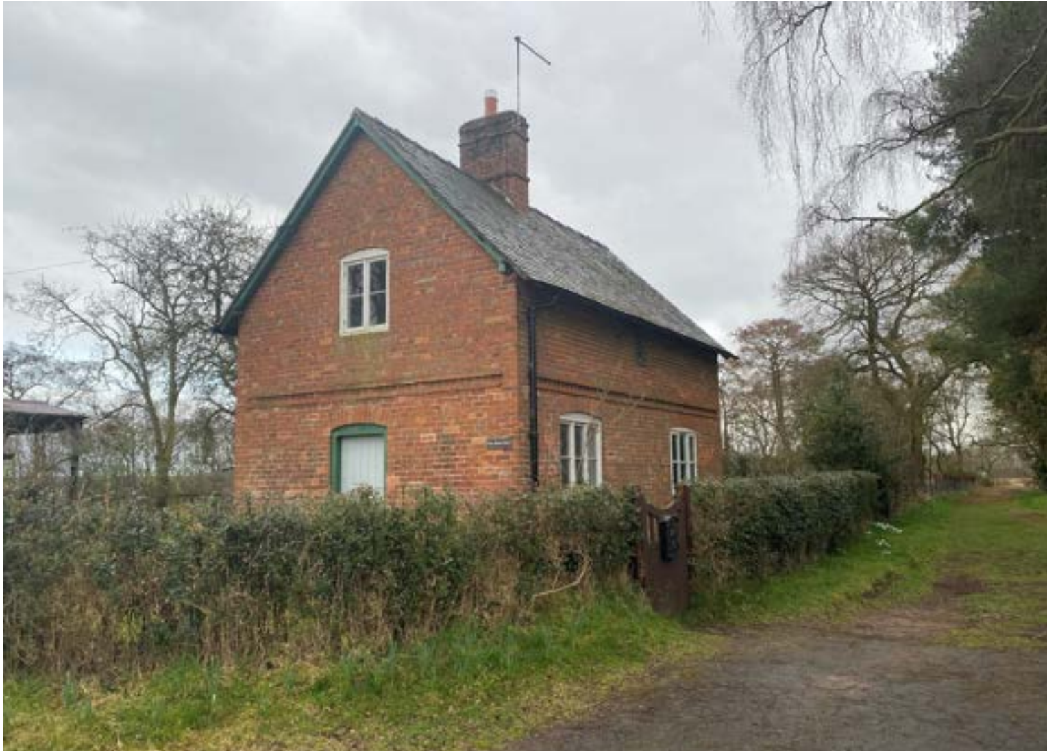
Figure 7 - The Site - northwest/southwest elevations.
