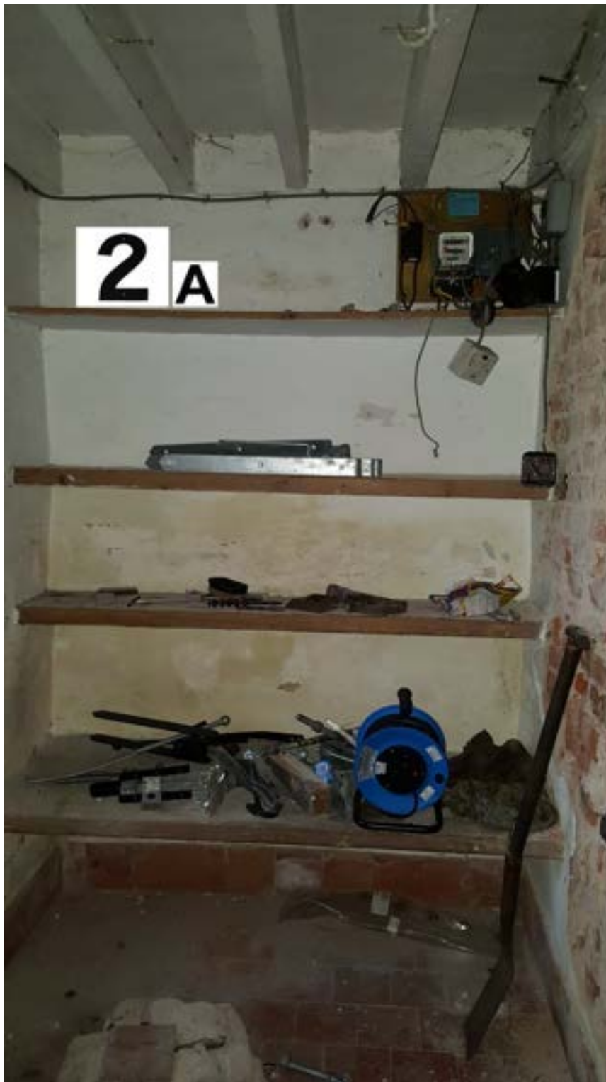
Figure 16 – Pantry shelves which have been lost as part of works already carried out. Photo taken from photographic survey discharged under P/2019/0904.
