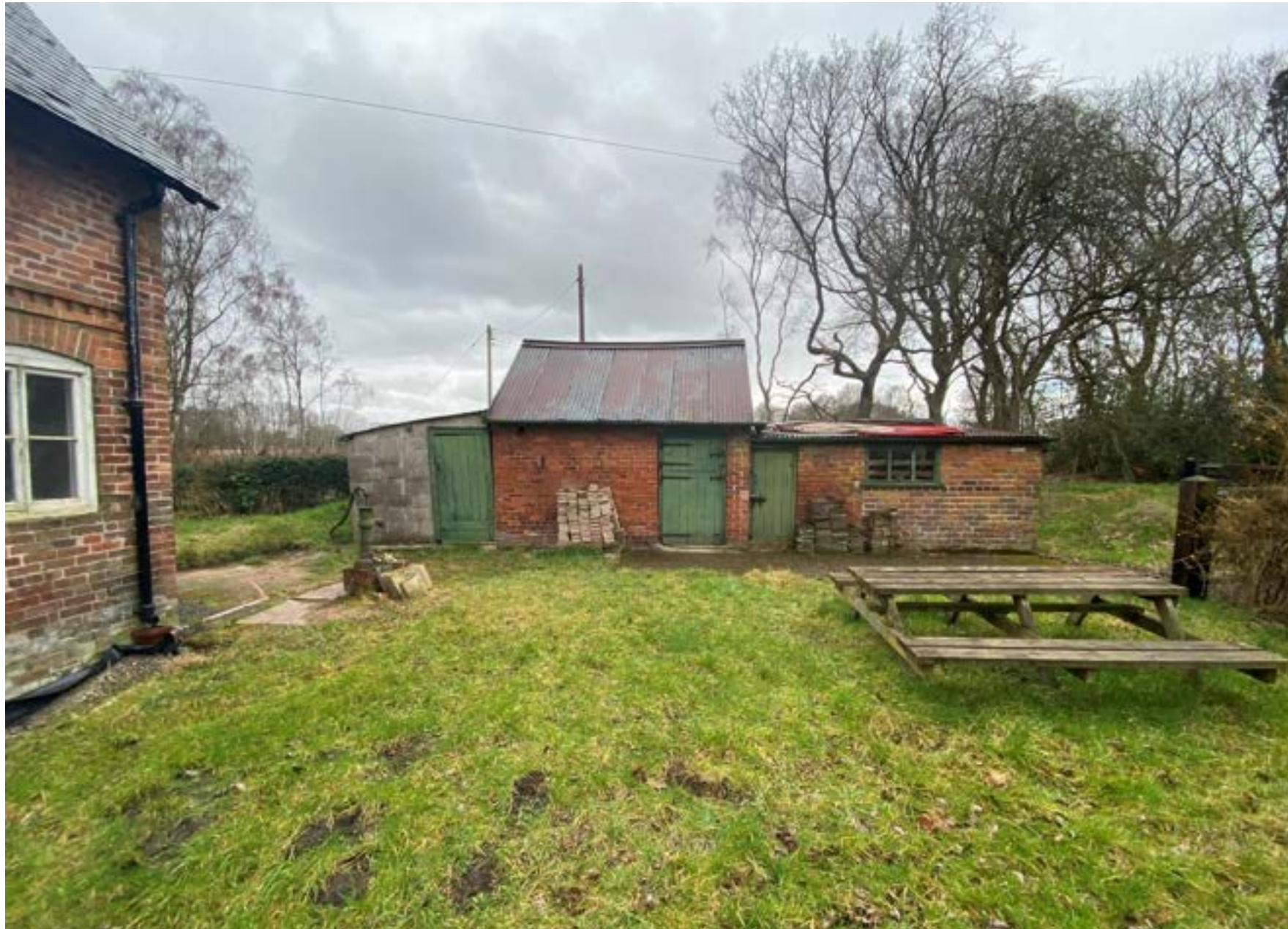
Figure 19 - The most historically significant of the outbuildings. Map regression shows a structure in this area.
