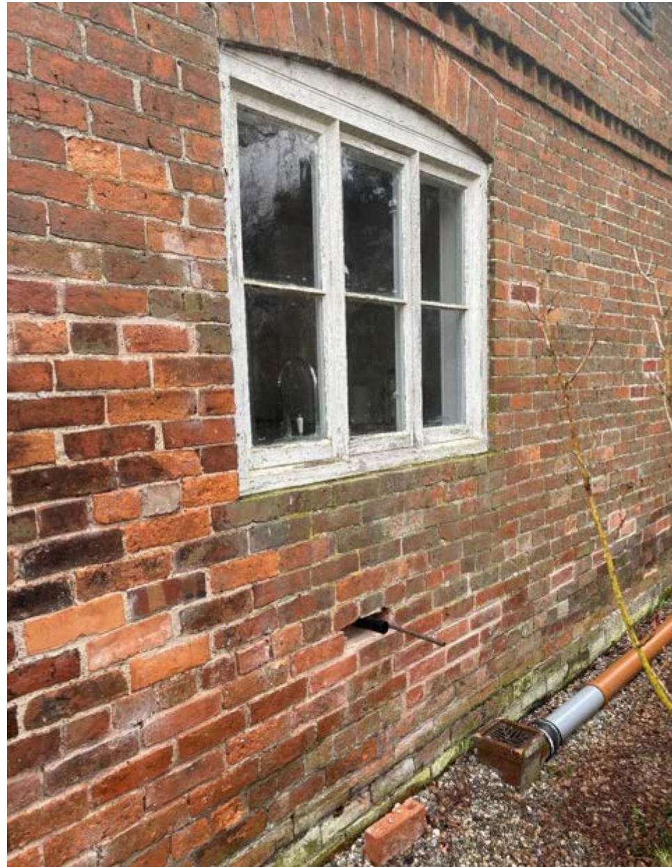
Figure 24 - Removal of brickwork and installation of piping. Purpose is unknown.
