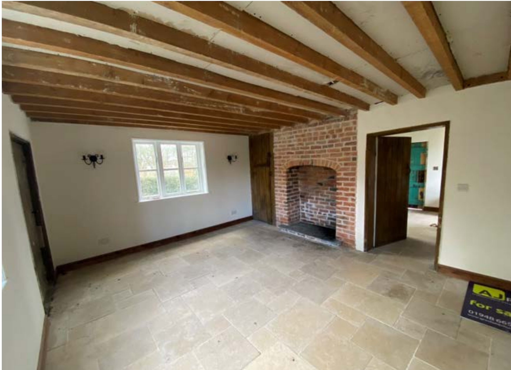
Figure 11 – Main living space within the Site. The significant fireplace is visible, as is the newly installed skirting boards.
