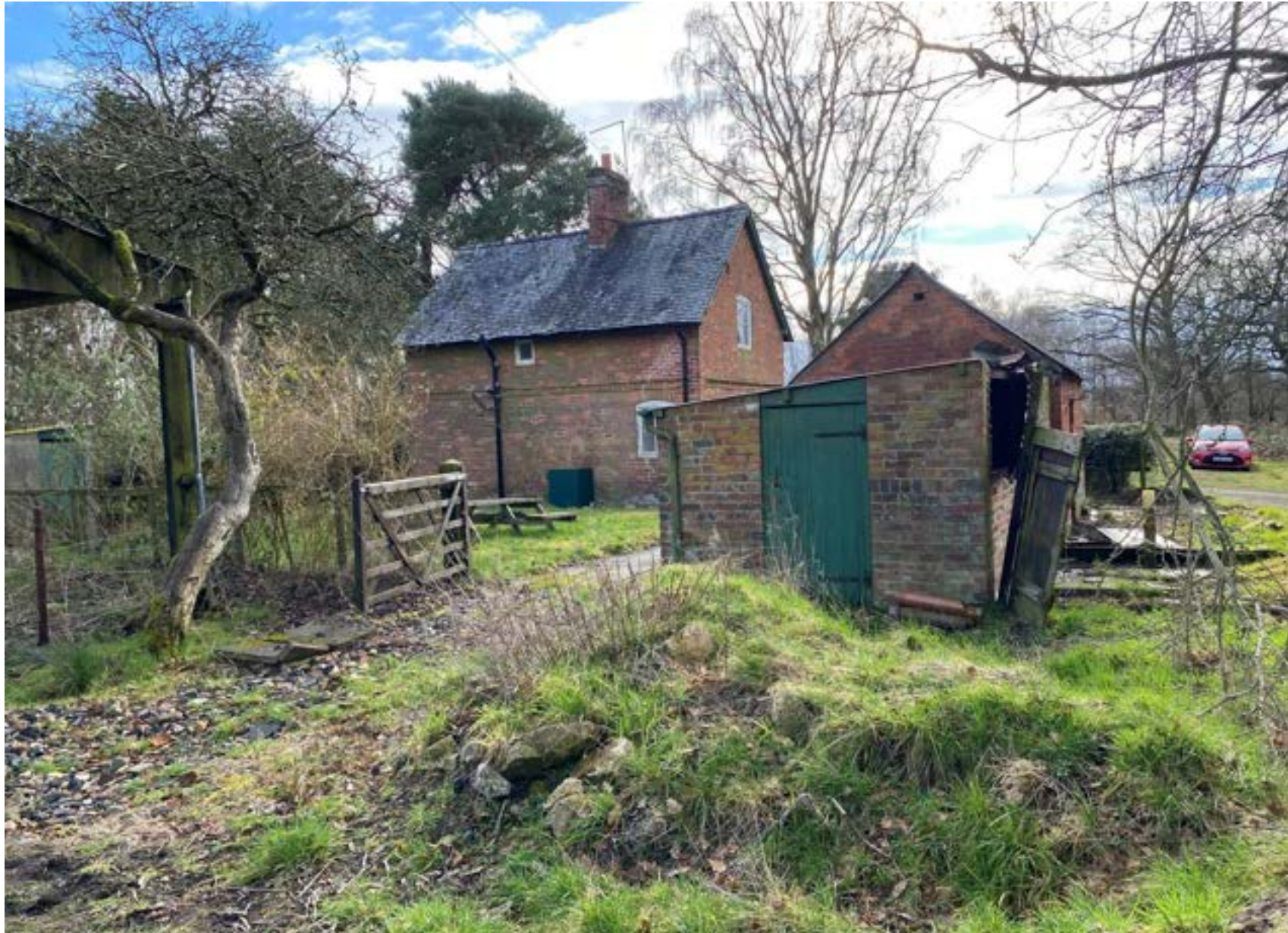
Figure 22 - Greater contextual view of the Site taking in all outbuildings and the main dwelling.
