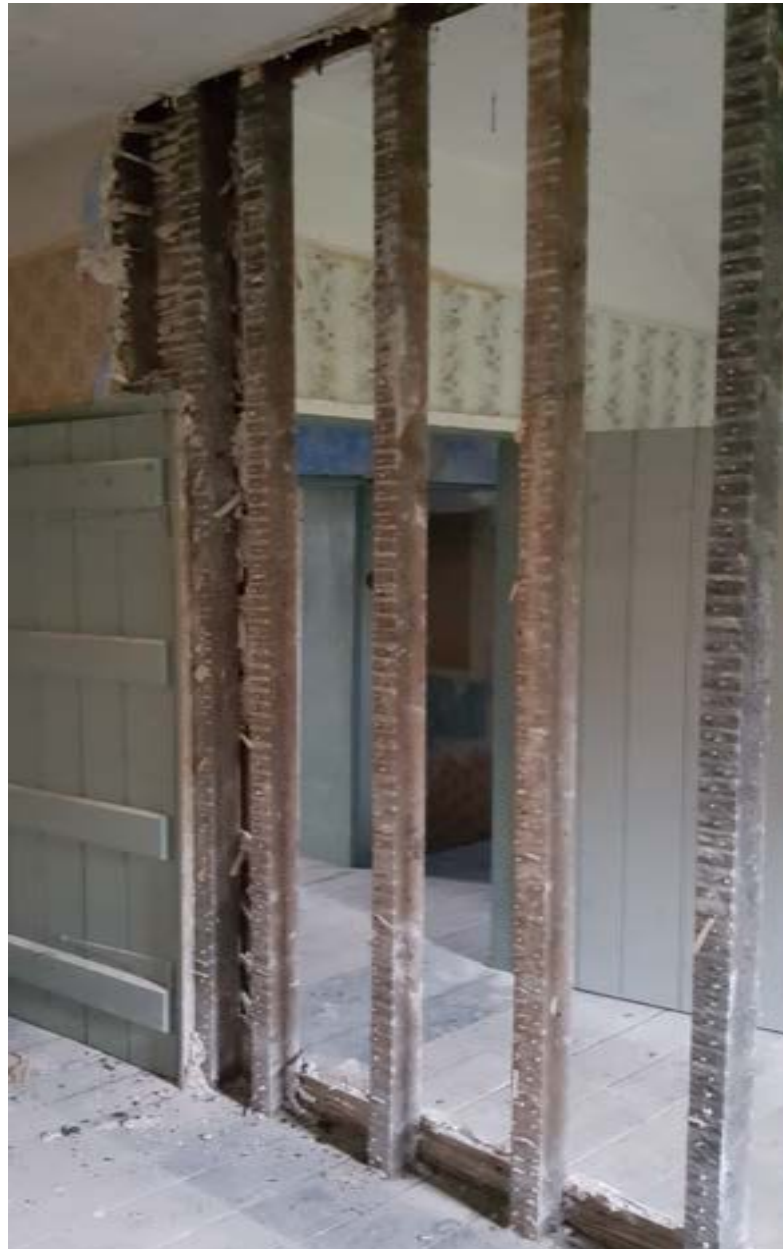
Figure 18 - Photo showing the pre-existing form of the wall separating bedroom two from the bathroom. Photo taken from photographic survey discharged under P/2019/0904.
