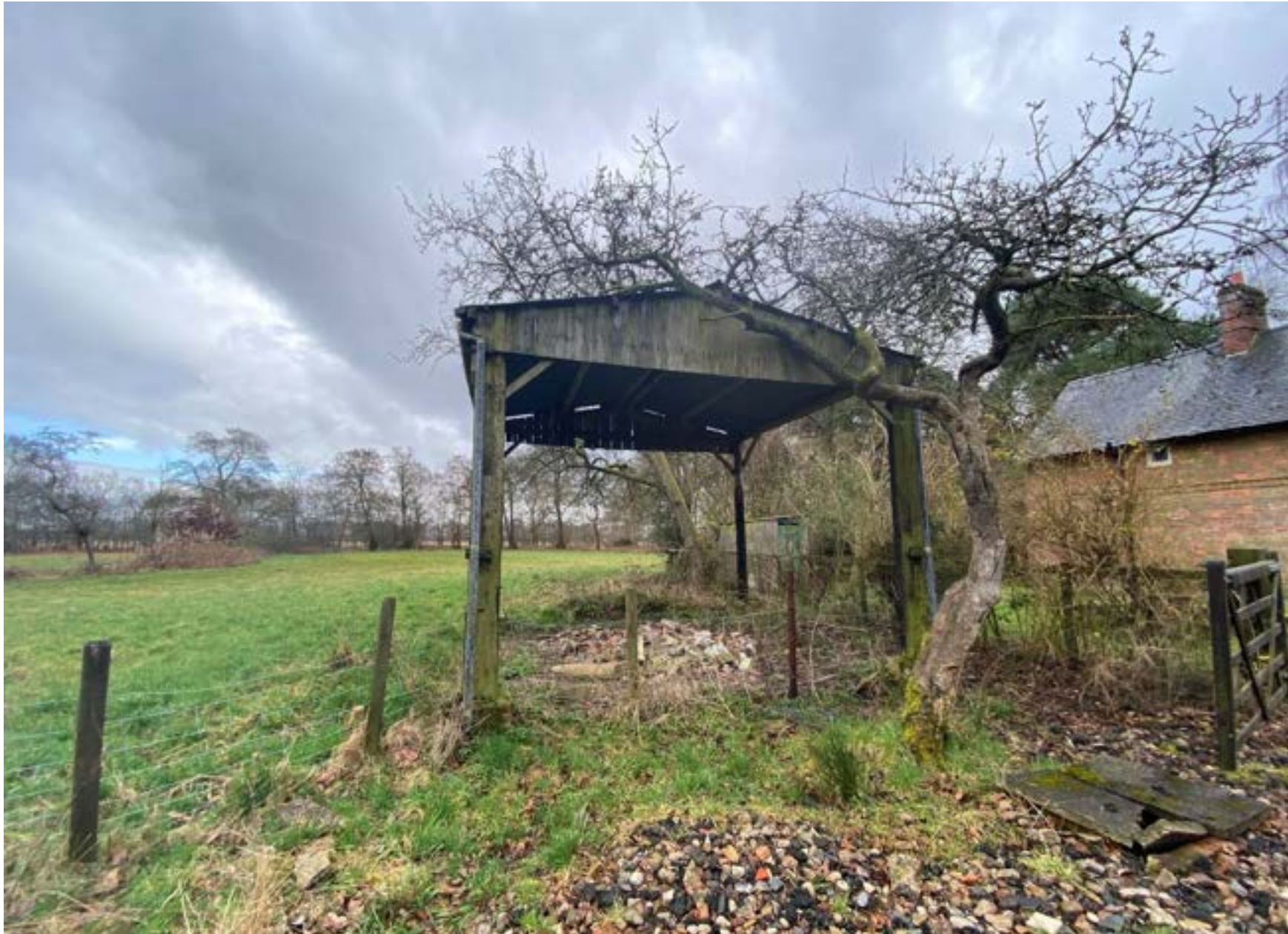
Figure 21 - Timber Dutch-barn structure on the Site's edge.
