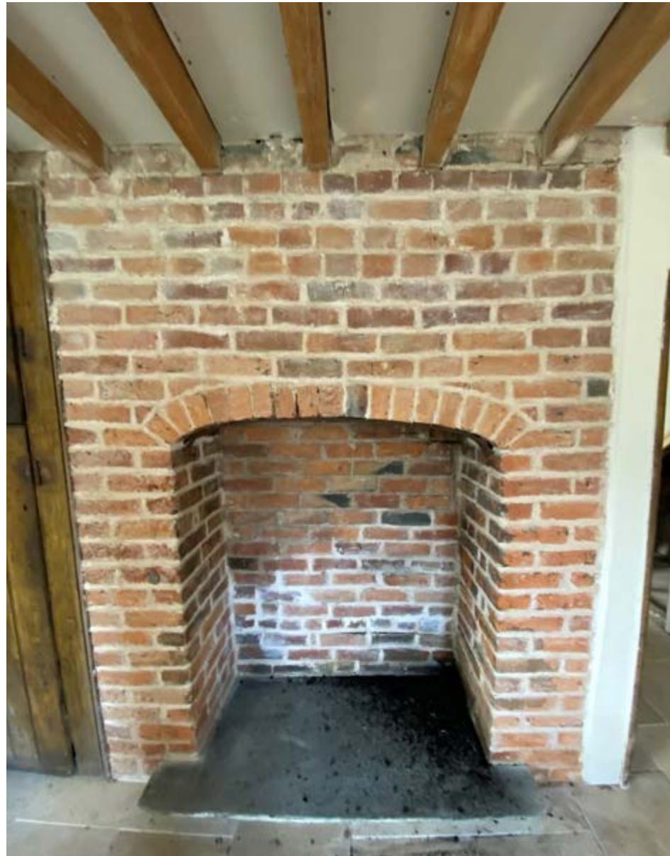
Figure 12 - Closer view of the fireplace.
