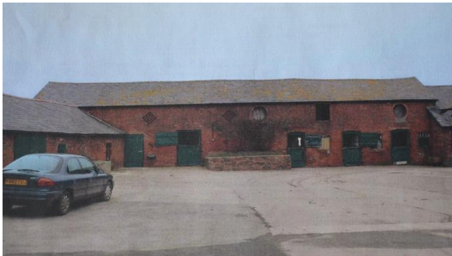
Pl.2: Late-20 th century view of the North Range or Stables, with the West Range to the left.
