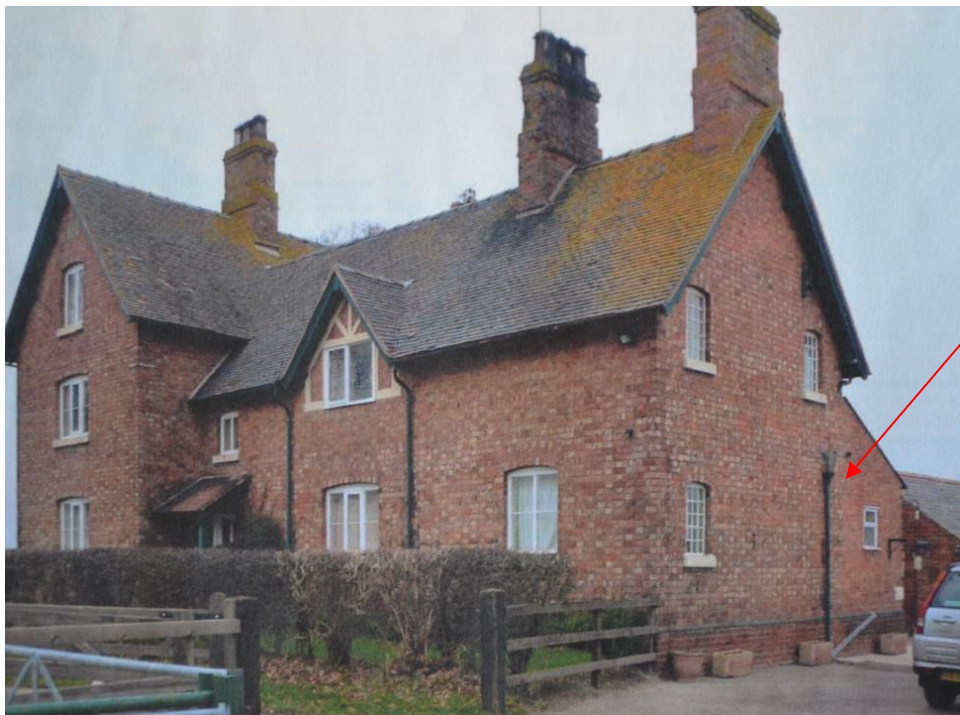
Pl.1: Late-20 th century view of the farmhouse from the south-east. The junction between the original build and the later lean-to with its different coloured brick and plinth is arrowed. Further to the right is the gable end of the West Range.
