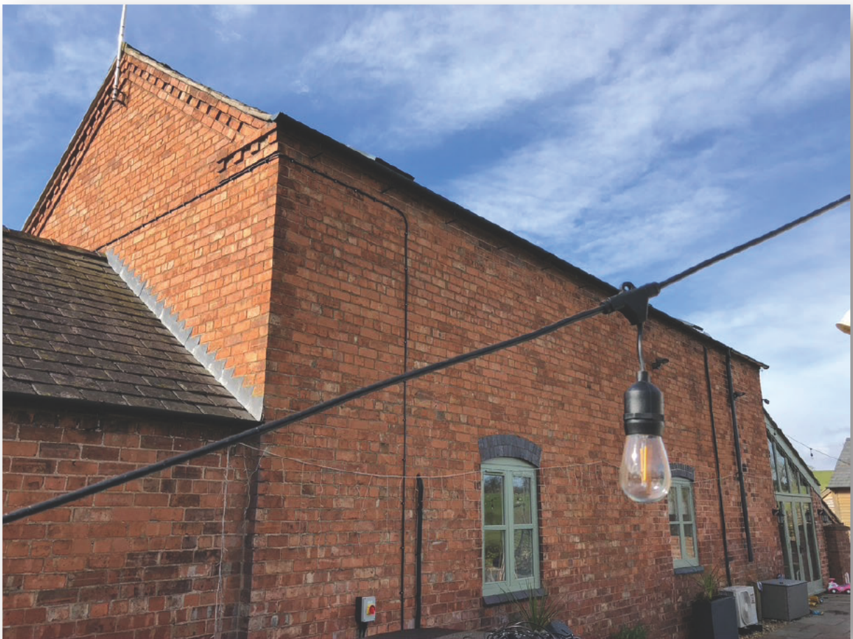
PHOTO 1: North elevation of dwelling with glazed opening in background
