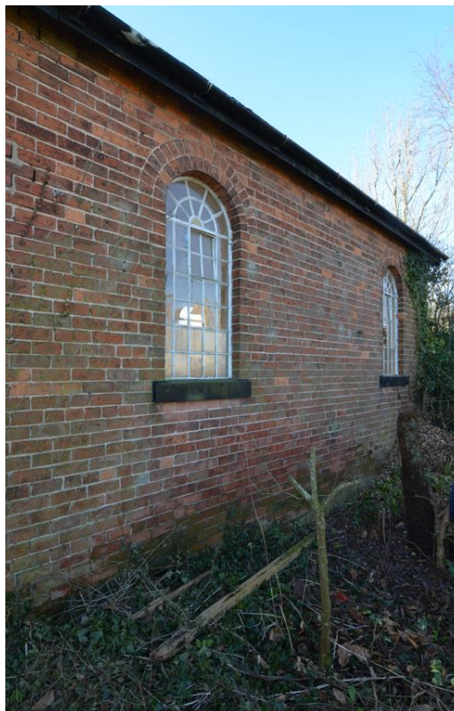
Pl.5: The rear elevation of the original Chapel.
