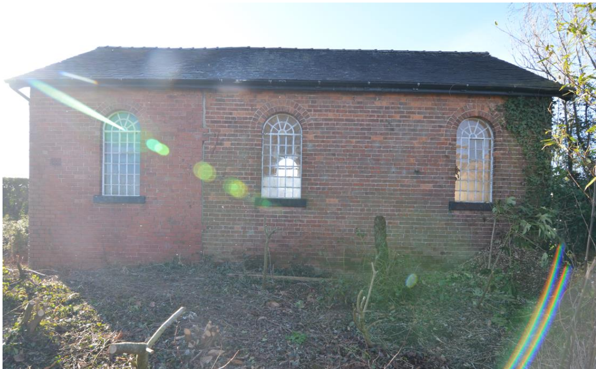
Pl.8: The rear elevation of the chapel, with the extension to the left.
