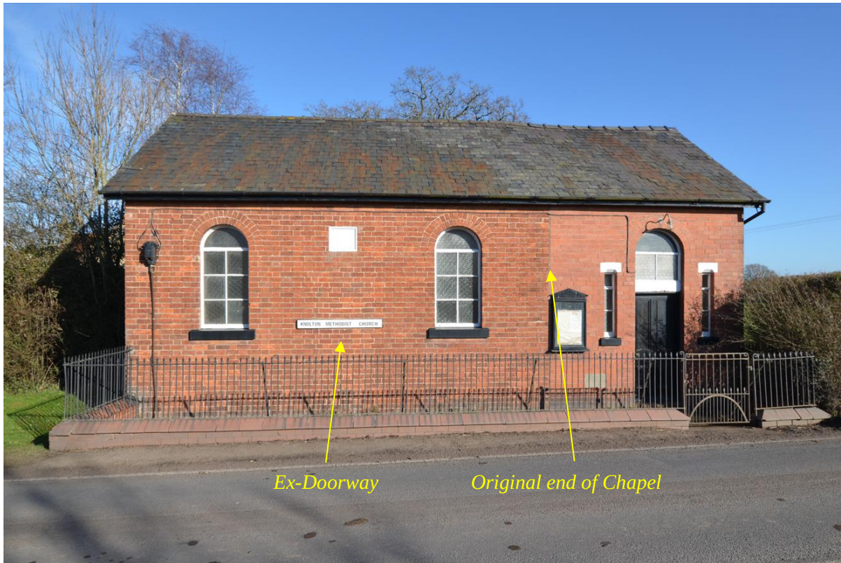
Pl.4: The front elevation of the Chapel.
