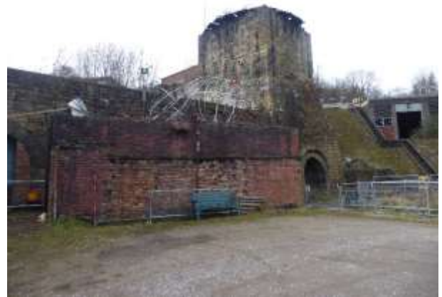
PHOTO 4.6. FRONT WALL AND BLAST FURNACE.
