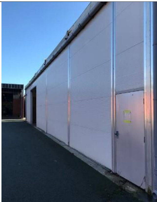
Photo 3 – showing an example of a completed warehouse with a metal frame flush with the ground and PVC walls and roof
