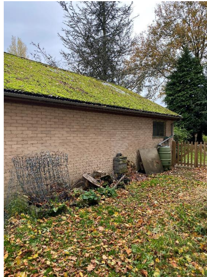
West elevation with concrete hardstanding in front of the gates to the garden.
