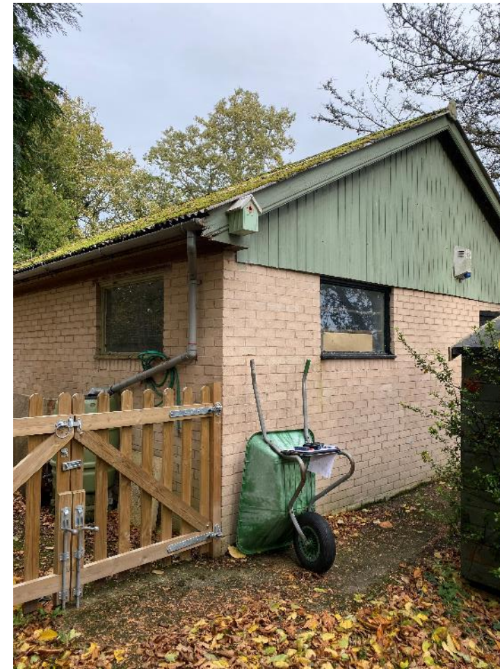
SW corner of the garage with concrete hardstanding wrapping round to the west.
