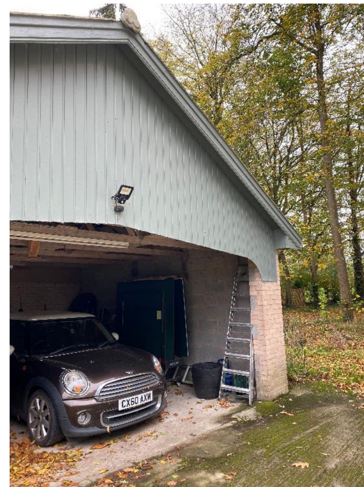
Front elevation of the garage.
