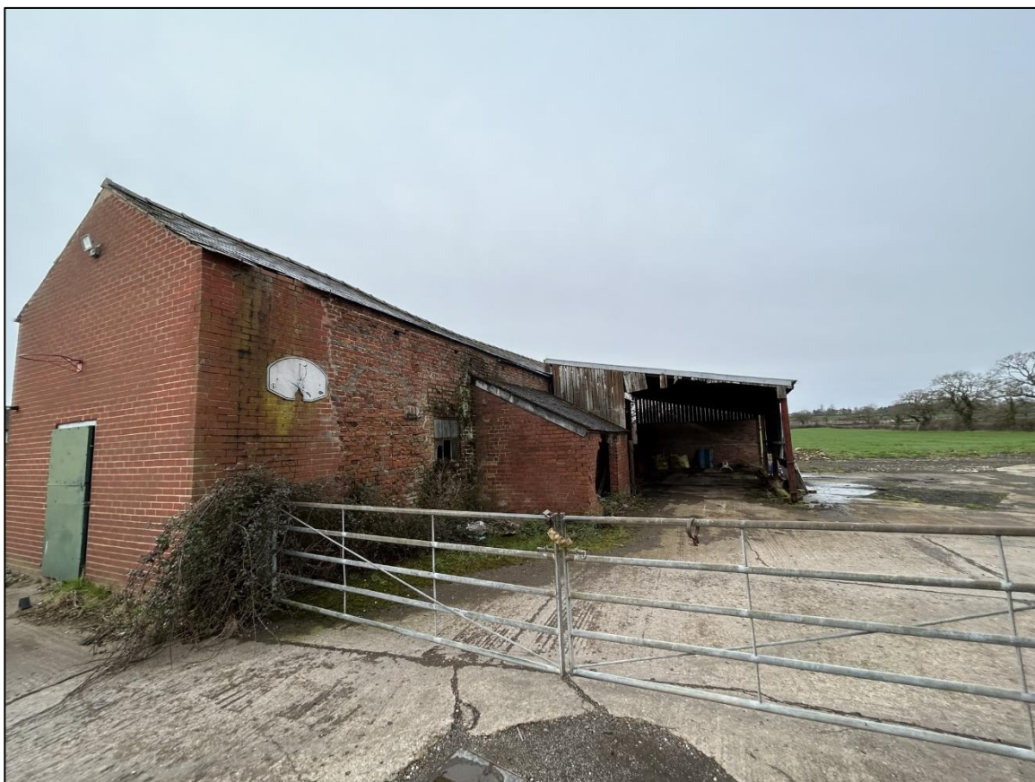
Plate 3 – The northern elevation of B1, with the timber built lean to present
