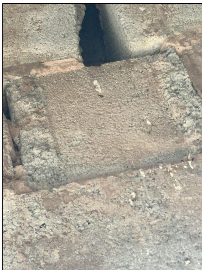
Plate 20 – Closer angle of PRF, note clear access to cavity
