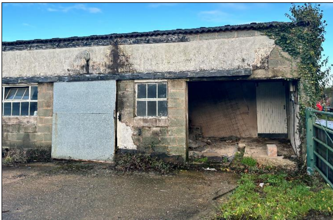
Plate 15 – Southern elevation of B2
