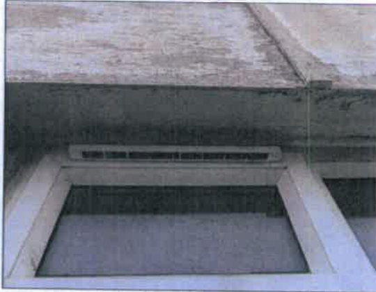
Plate 13. Ply barge board absent (pitched roof)
