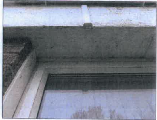
Plate 12. Ply barge board absent (flat roof)
