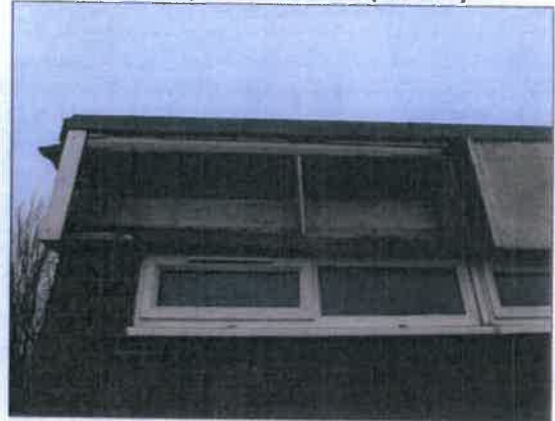
Plate 14. Flat roof covering flush to fascia boards
