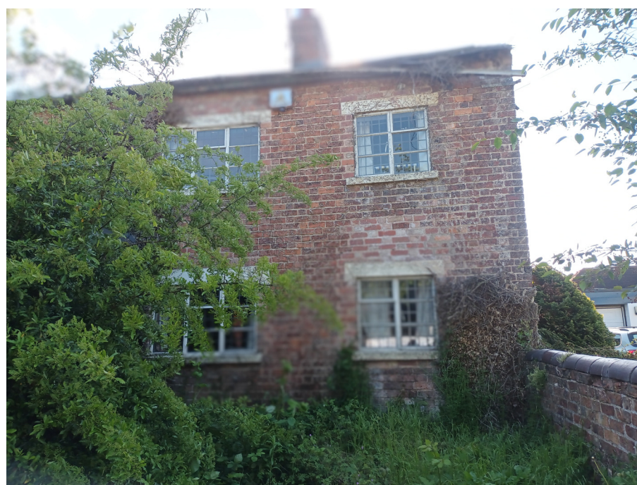
End Front Elevation Showing varying brickwork
