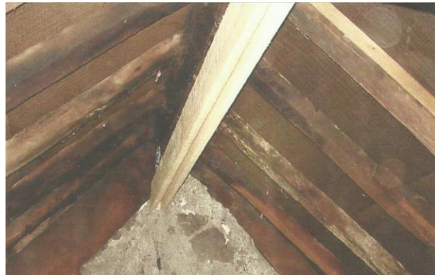
Figure 11: Example of crevice box in a loft void.
