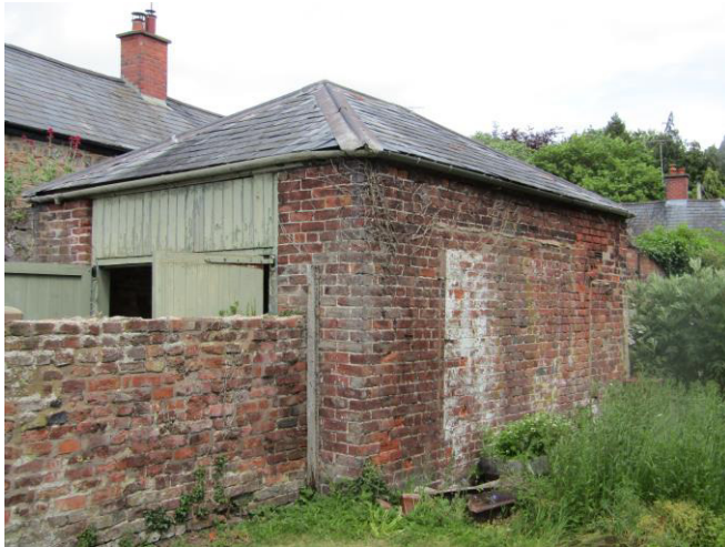
Photo 1: Brick garage to South of building.
