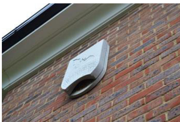
Figure 9: Schwegler (1WQ) bat box fitted to wall.
