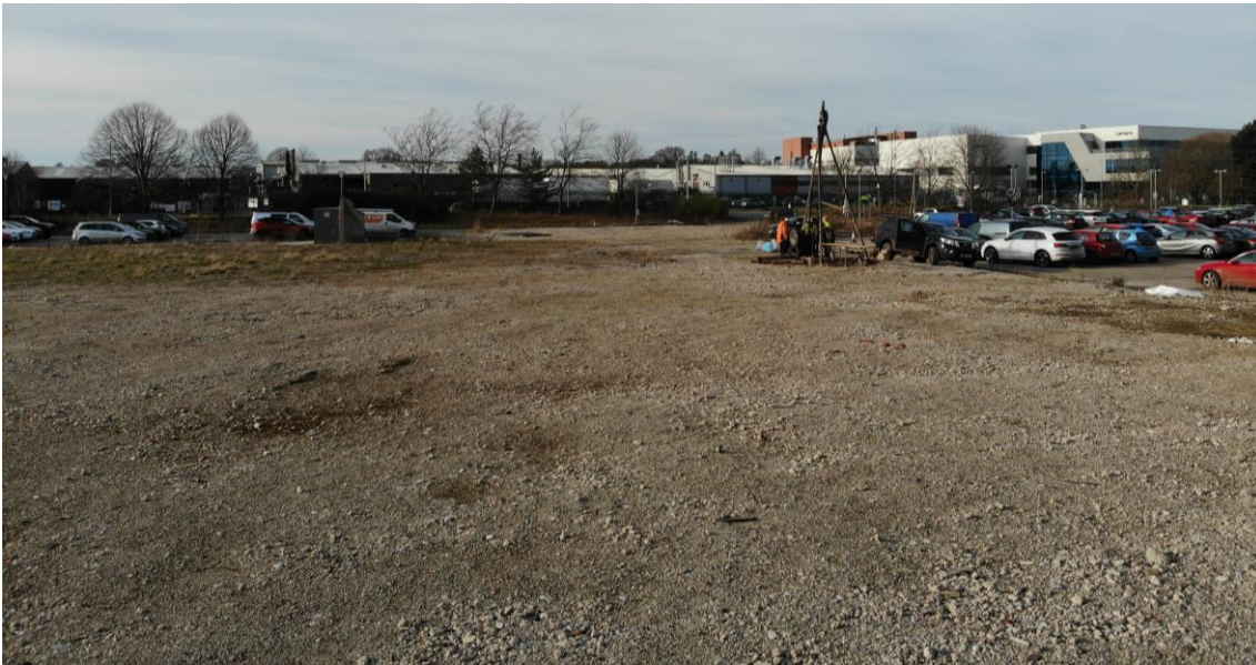
Figure 5 – existing site, looking northwest towards main Ipsen Campus
