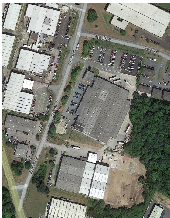
Figure 19 - Proserve building pre-demolition
