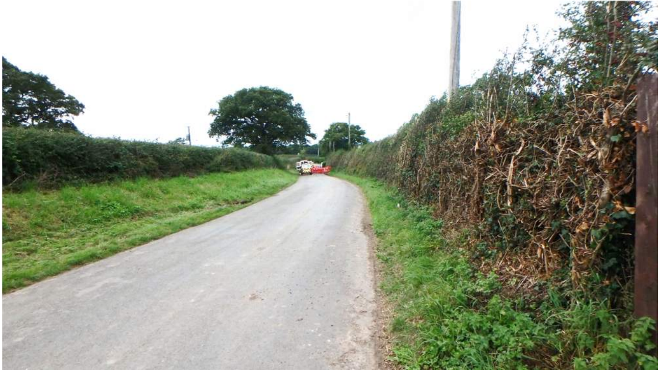
PHOTOGRAPH 3 Road channel in a westerly direction from the existing access
