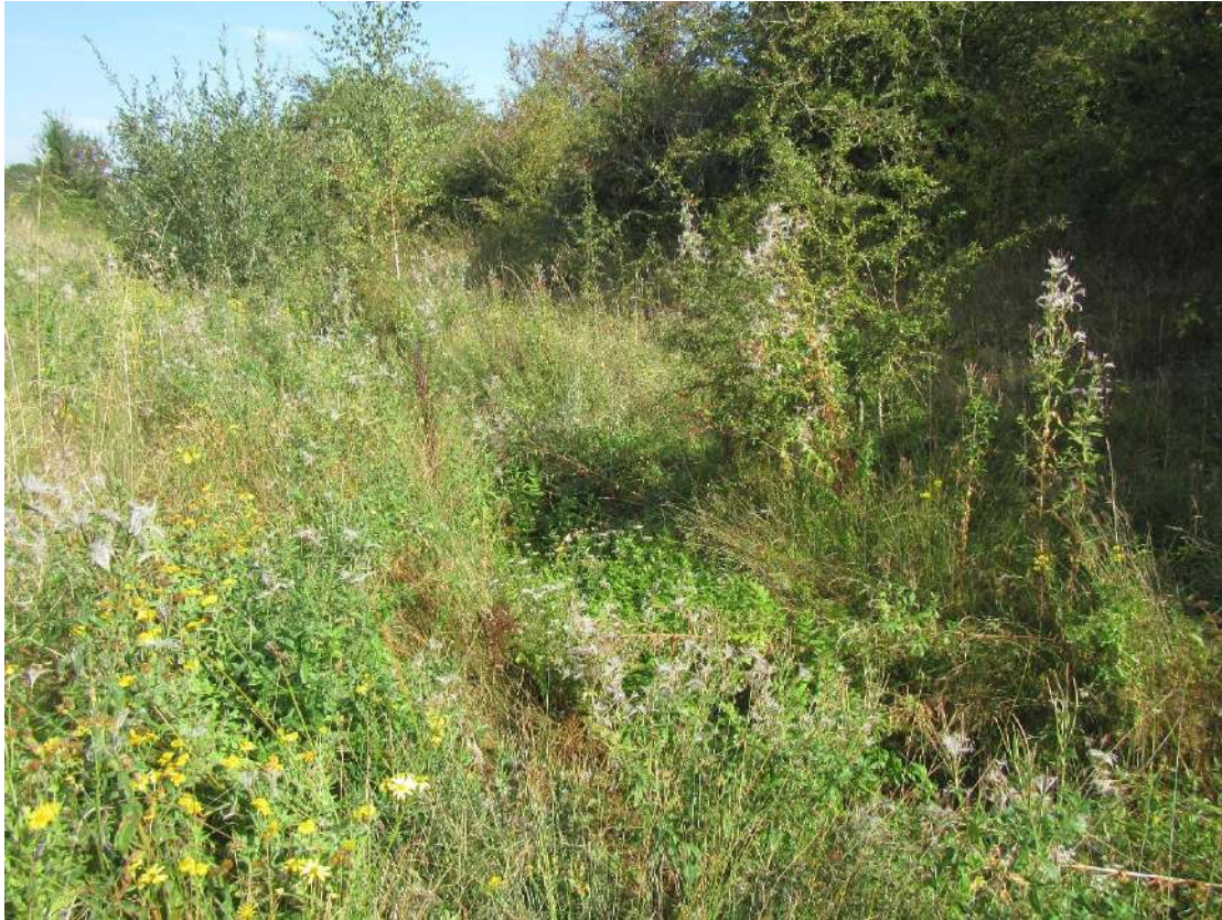
Photograph 19 – The ditch along the eastern site boundary is heavily vegetated and is being encroached by scrub.
