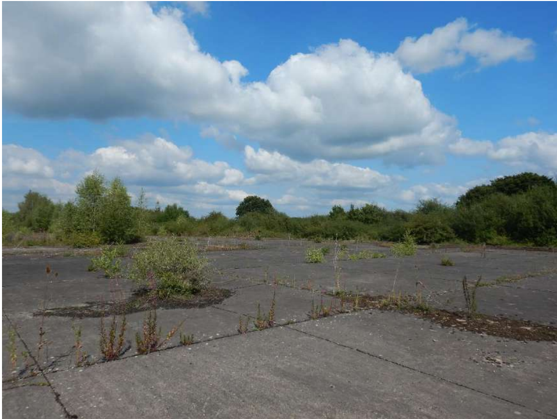
Photograph 24 – Example of large area of intact hardstanding in the south-eastern section of the site.
