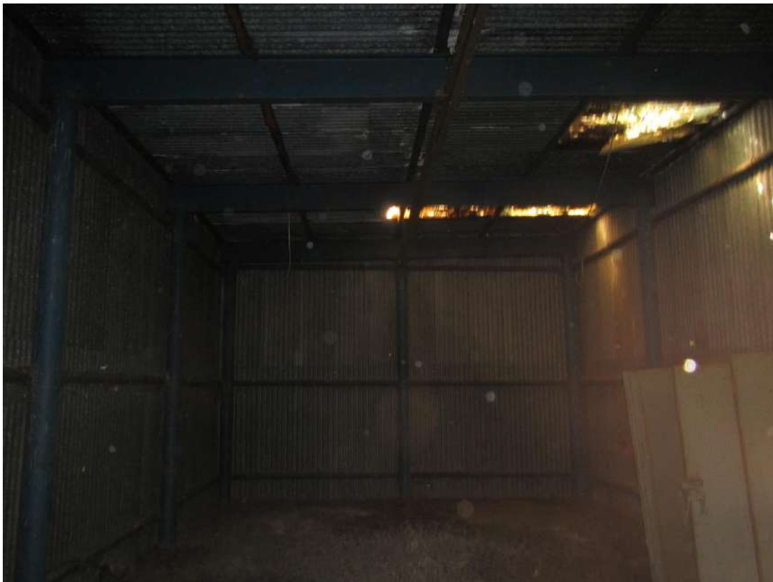
Photograph 30 – Internal view of Building 2.
