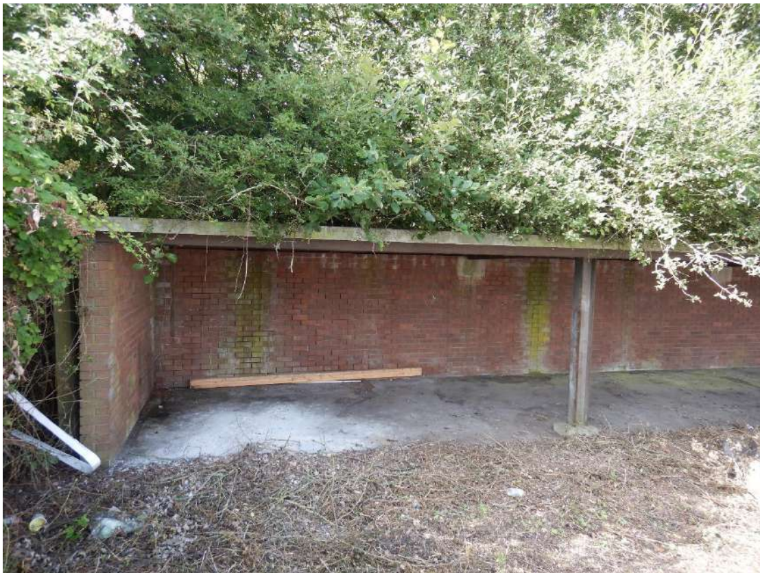
Photograph 28 – View of Building 1.
