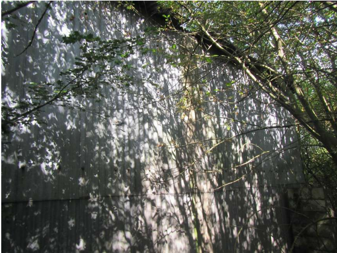
Photograph 29 – External view of Building 2.
