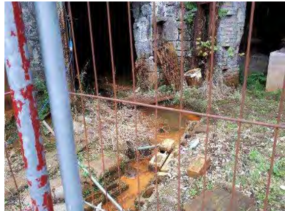
Foundry Adit discharge to Foundry Adit Drain
