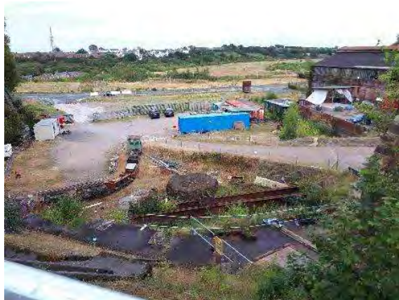
View E over southern end of lower Central Heritage area area
