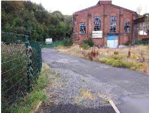
View W from southern spine road access over Car Park with Central Heritage area beyond; Machine Shop frontage
