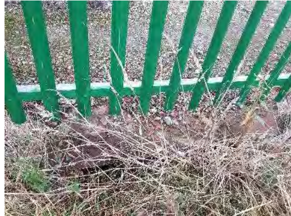
Covered drain containing Foundry Adit drain at southern boundary to central heritage area
