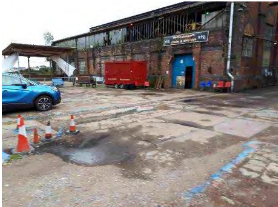
View S over Central Heritage Area, lower level; Machine Shop
