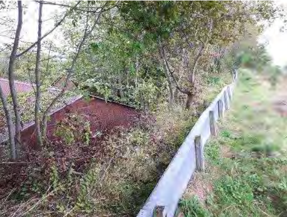
View E along southern boundary Blast Pit area with Haul Road (past ruined colliery buildings)
