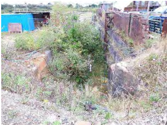
Open ditch containing Foundry Adit drain in Central Heritage Area
