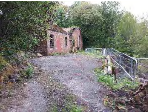
View E. up track to ruined Blast Pit colliery buildings
