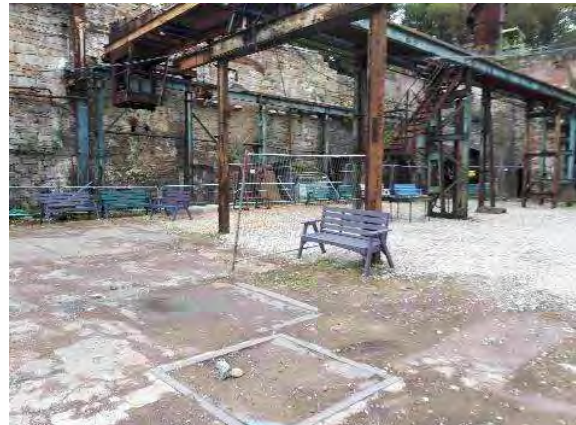
View N over Central Heritage Area, lower level; Forge Area
