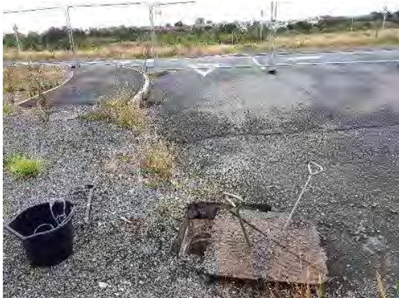
Manhole cover to Foundry Adit drain at site boundary
