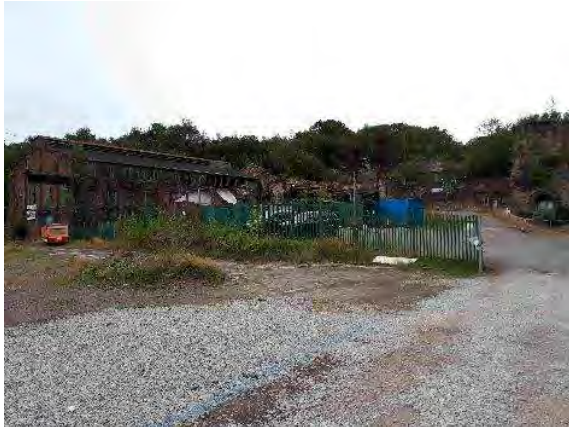
View SW from northern spine road access over Car Park with Central Heritage area beyond
