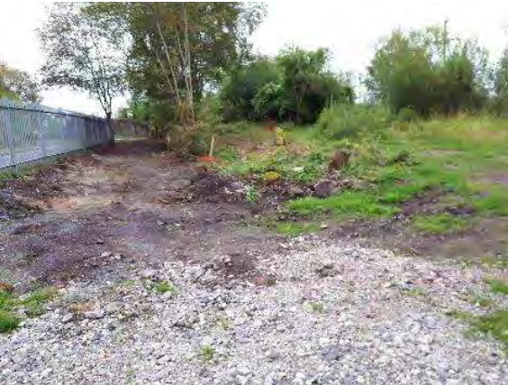
View E over lower Blast Pit area
