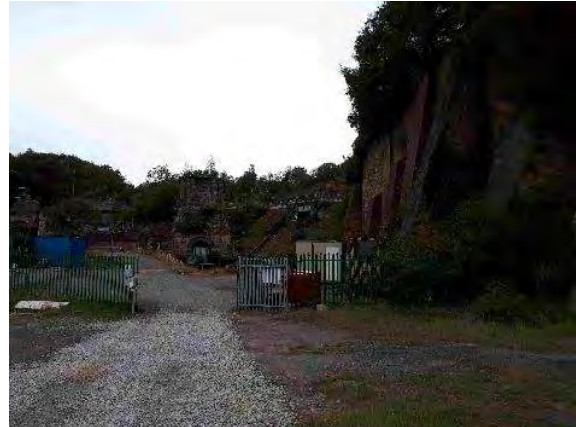
View W from northern spine road access over Car Park and entrance gate with Central Heritage area beyond; retaining walls form northern boundary with adjacent Enterprise Centre
