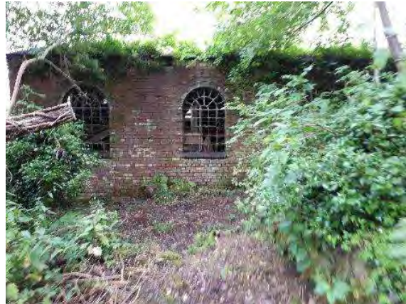
Ruined Blast Pit colliery buildings
