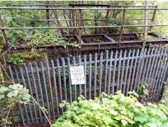
Western Blast Pit shaft
