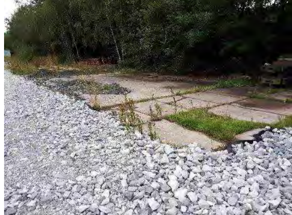
View N from over central upper Duck Pond area concrete slabs past wooded bank down to lower Duck Pond area
