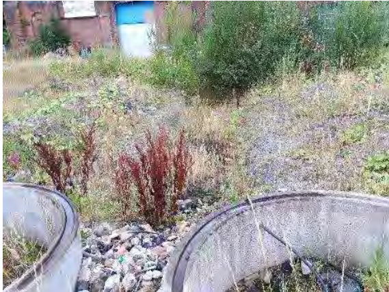
Open ditch containing Foundry Adit drain in Car Park area
