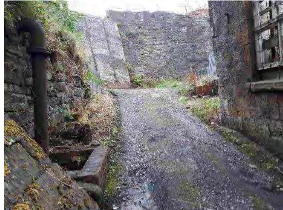
View W up access ramp between lower and middle Central Heritage areas past Forge
