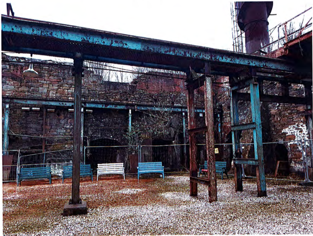
Photograph 8 Adit inside right had entrance
