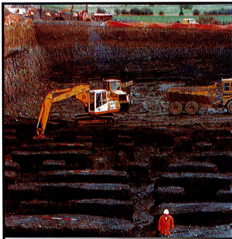
Example of pillar and stall workings exposed in an opencast
