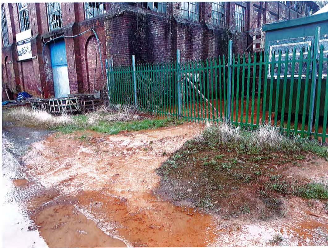
Photograph 1 Mine water discharge from adit
