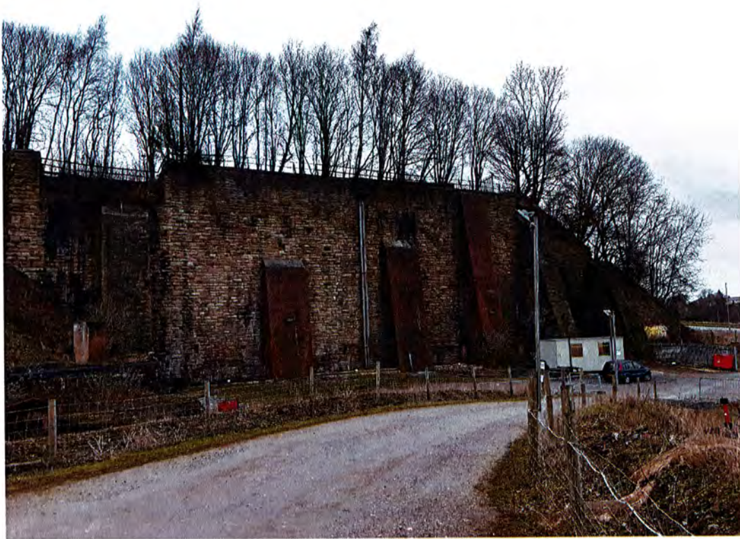
Photograph 6 Retaining structure on northern site boundary
