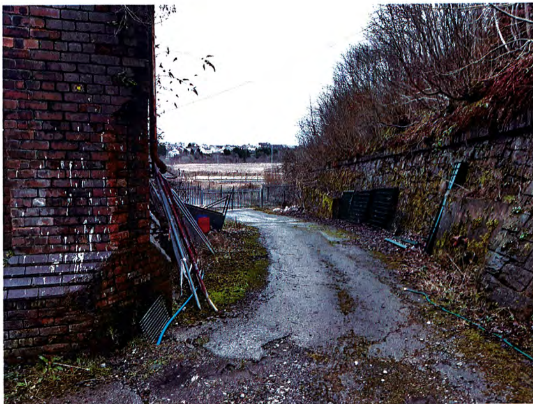
Photograph 11 Path on southern site boundary
