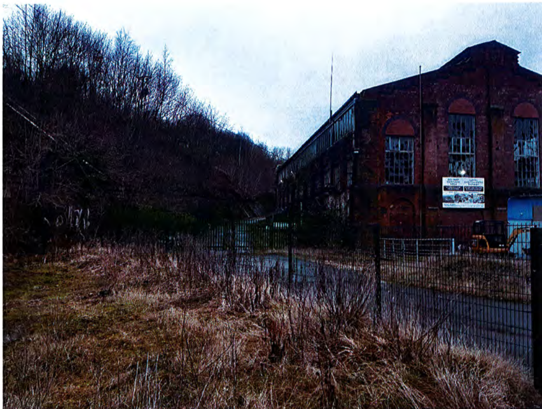
Photograph 3 Southern side of site showing ground level rising rapidly to the south
