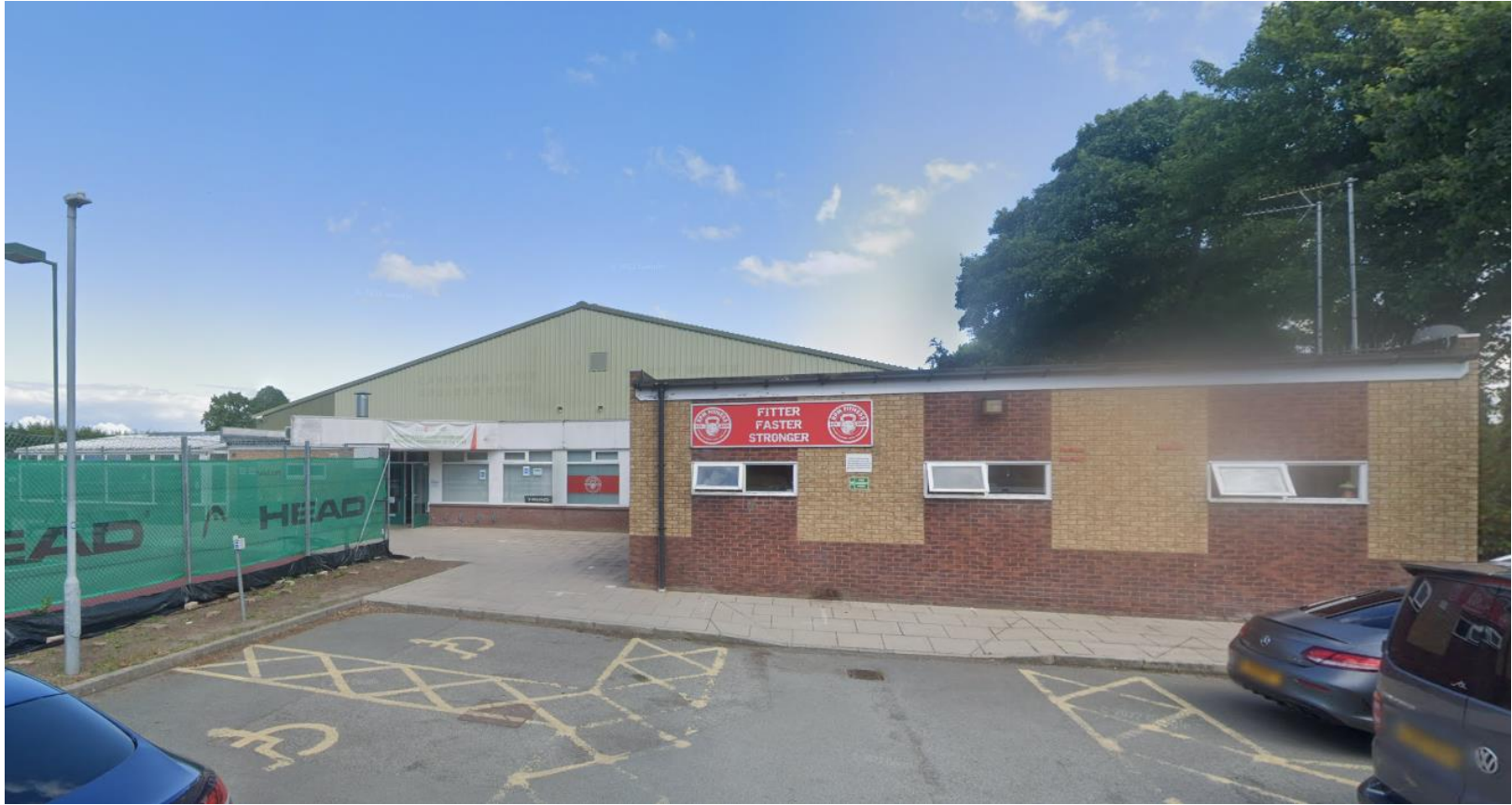
External View of Frontage from Car Park
