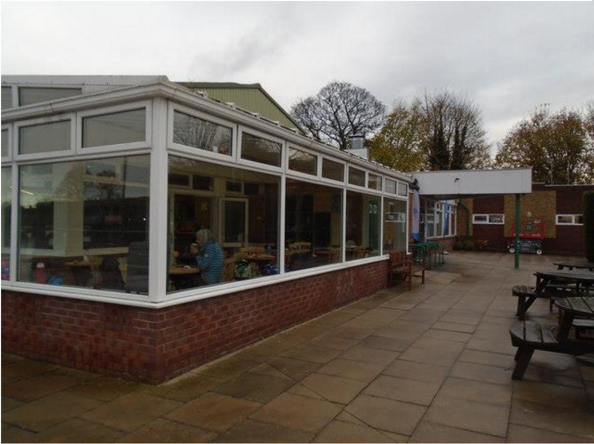
External View of Corner Conservatory Extension
