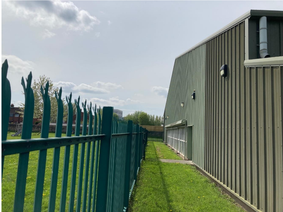
External View of Portal Frame South Gable
