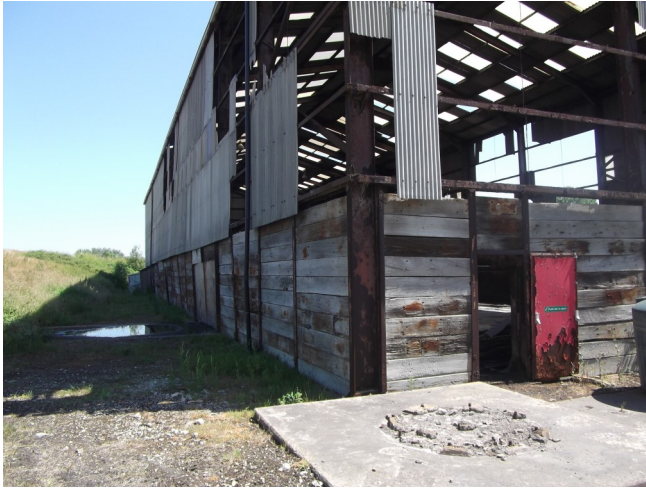
The storm ravaged South Western corner of Unit 3 and its gable end. Note the sleeper walls.
