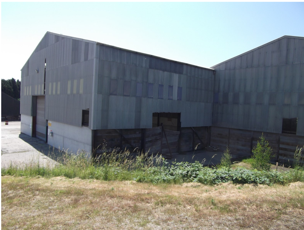
The Northern elevation of Unit 5 and the North Eastern elevation (the gable end) of the adjoining Unit 3 taken from atop The Hill.
