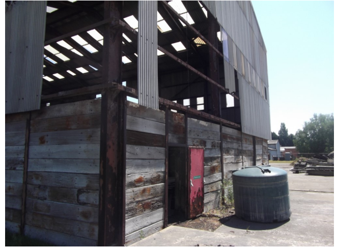
The storm ravaged South Western corner of Unit 3 and its gable end. Note the sleeper walls.
