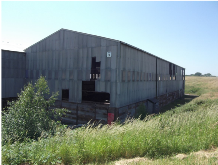
The North Eastern elevation of Unit 3 taken from The Hill.
