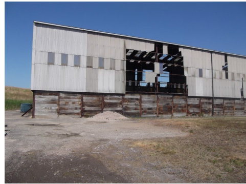
Above and below shows the storm damaged South facing elevation of Unit 3 leading to Unit 5.
