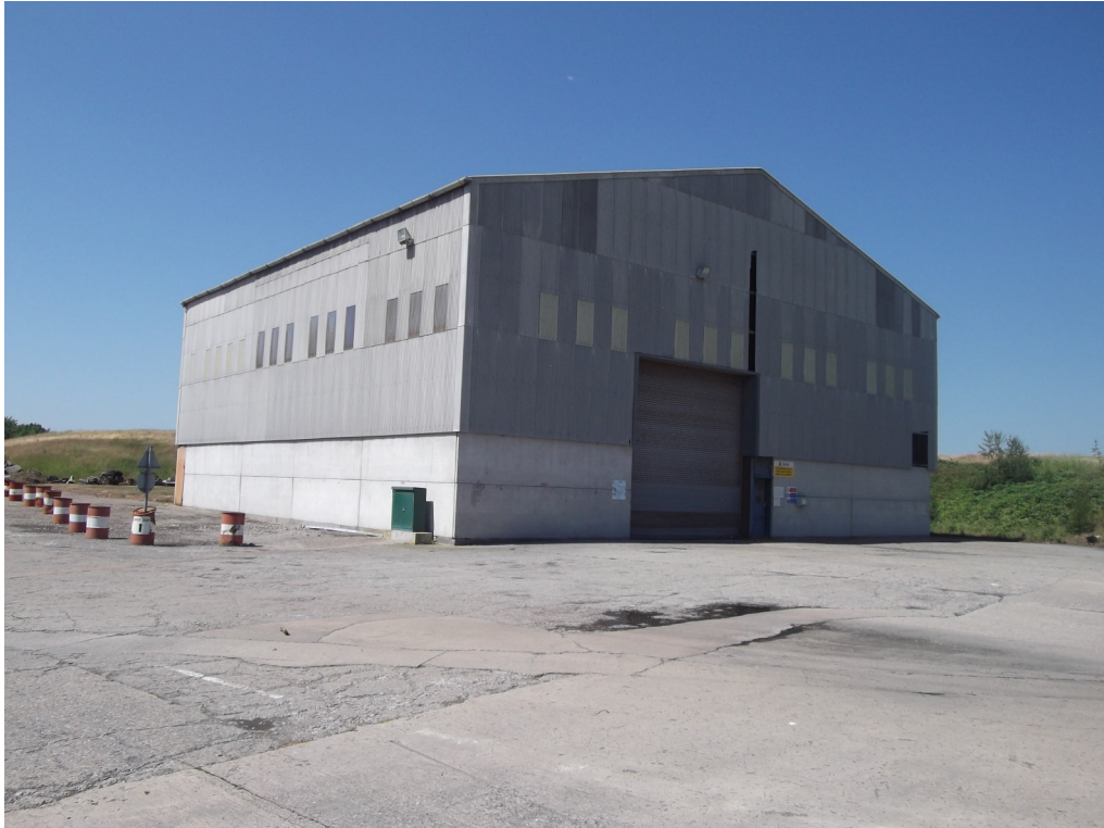
The North Eastern elevation of Unit 5 taken from the roundabout.
