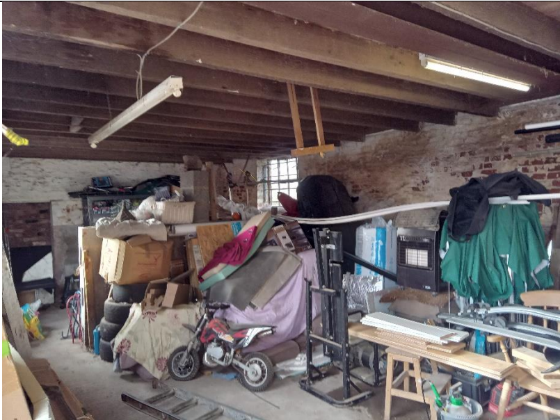
B1 – interior – ground floor
