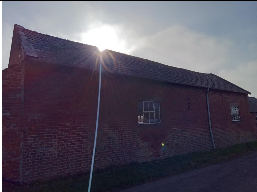
B1 – northern elevation – intact tiles
