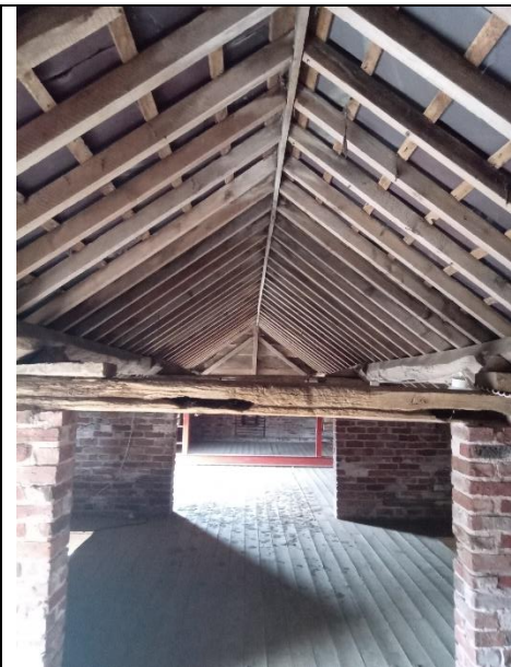
B1 – interior – roof void
