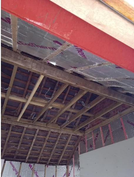
B1 – storage space 2 – undergoing refurbishment – (not part of the proposed development)
