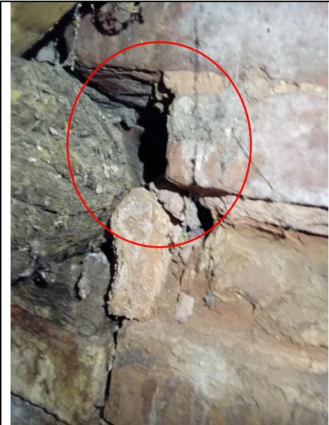
B1 – interior – roof void – crevice example
