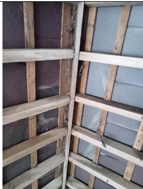
B1 – interior – roof void - unlined
