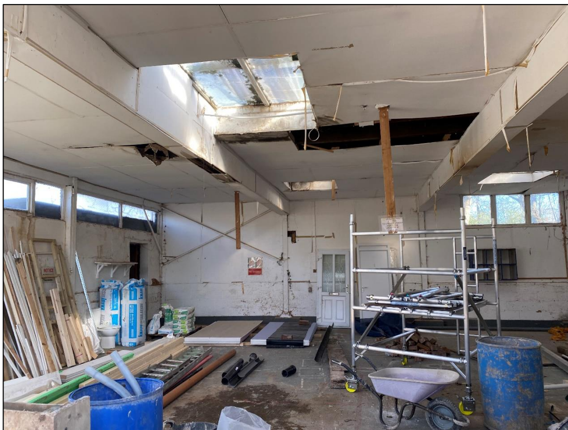
Plate 5 – Interior of B2
