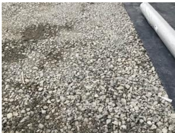
Sub grade prior to membrane installation
