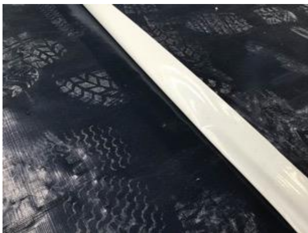
Sealed tape joint
