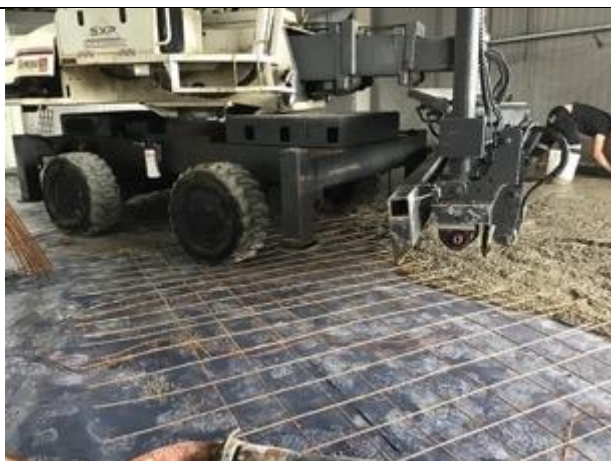
Laser screed on top of mesh / membrane
