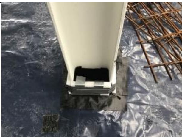
Sealed stanchion detail
