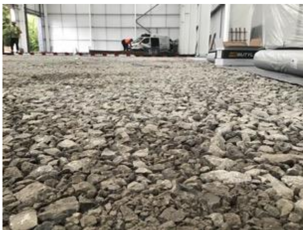
Sub grade prior to membrane installation
