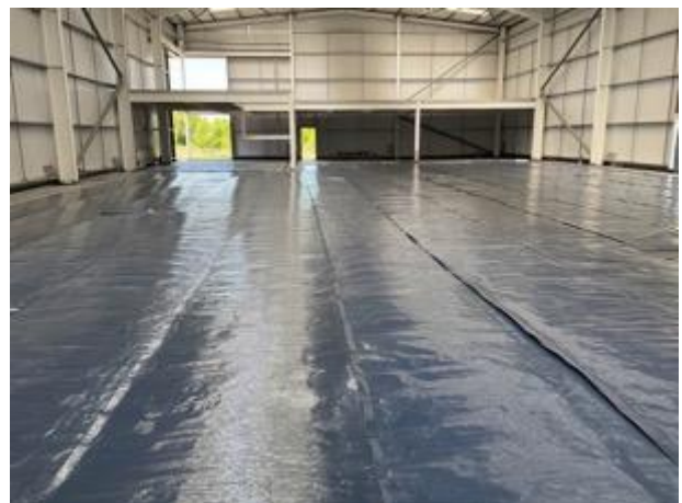
General overview opposite direction
