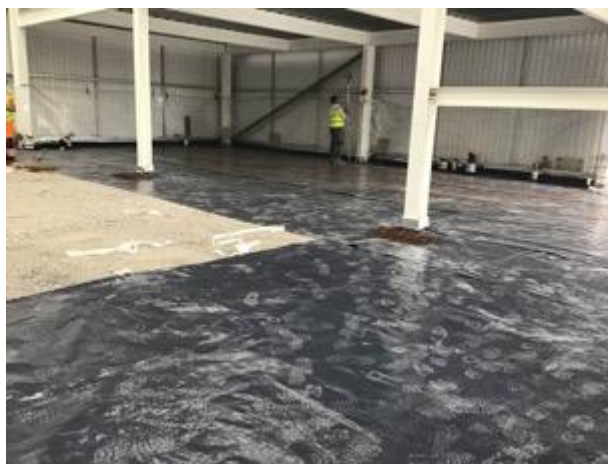
Unit 2 membrane installation
