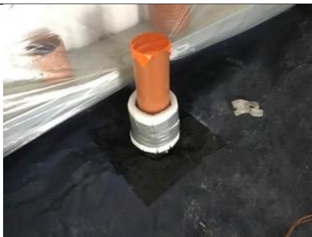
Sealed pipe penetration
