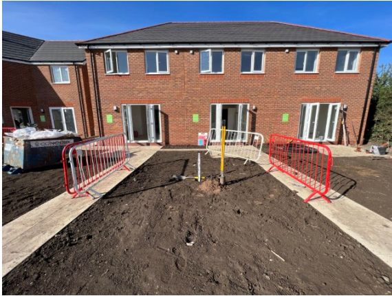
Photographs 4 & 5: Showing the depth of the inert cover and location of the validation hole within the rear garden of Plot 232 and the depth of inert cover achieved. Photographs taken 13 th September 2023.
