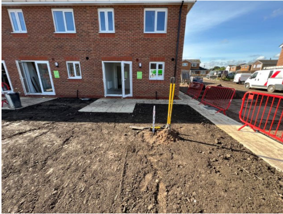
Photographs 13 & 14: Showing the depth of the inert cover and location of the validation hole within the rear garden of Plot 235 and the depth of inert cover achieved. Photographs taken 13 th September 2023.
