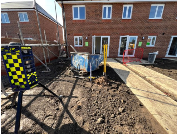
Photographs 19 & 20: Showing the depth of the inert cover and location of the validation hole within the rear garden of Plot 237 and the depth of inert cover achieved. Photographs taken 13 th September 2023.
