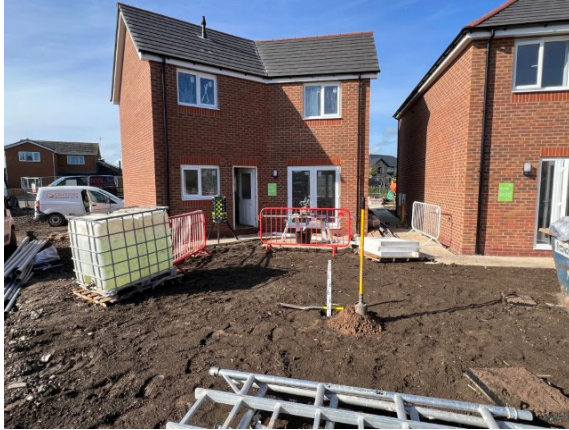
Photographs 10 & 11: Showing the depth of the inert cover and location of the validation hole within the rear garden of Plot 234 and the depth of inert cover achieved. Photographs taken 13 th September 2023.
