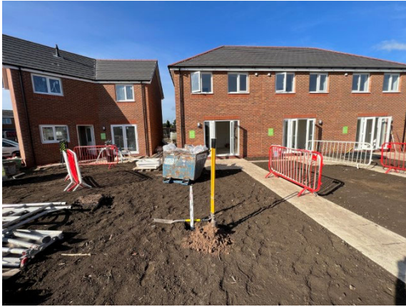
Photographs 7 & 8: Showing the depth of the inert cover and location of the validation hole within the rear garden of Plot 233 and the depth of inert cover achieved. Photographs taken 13 th September 2023.
