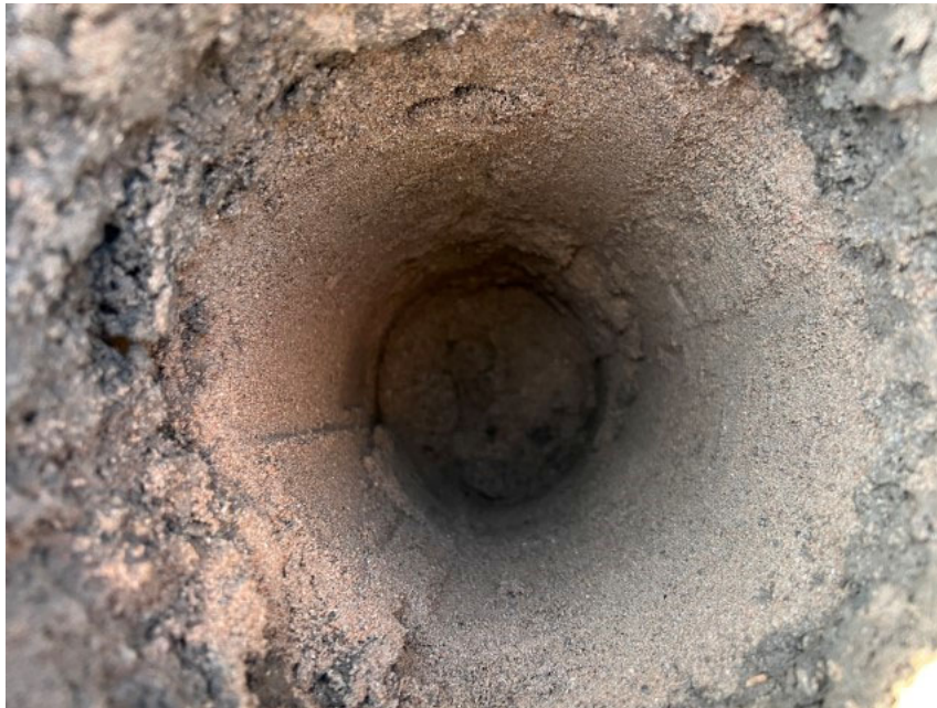
Photograph 15: Photograph shows the nature of the inert cover within the validation hole in the rear garden of Plot 235. Photograph taken 13 th September 2023.
