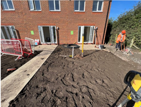
Photographs 1 & 2: Showing the depth of the inert cover and location of the validation hole within the rear garden of Plot 231 and the depth of inert cover achieved. Photographs taken 13 th September 2023.
