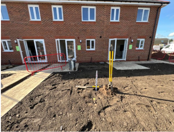
Photographs 16 & 17: Showing the depth of the inert cover and location of the validation hole within the rear garden of Plot 236 and the depth of inert cover achieved. Photographs taken 13 th September 2023.
