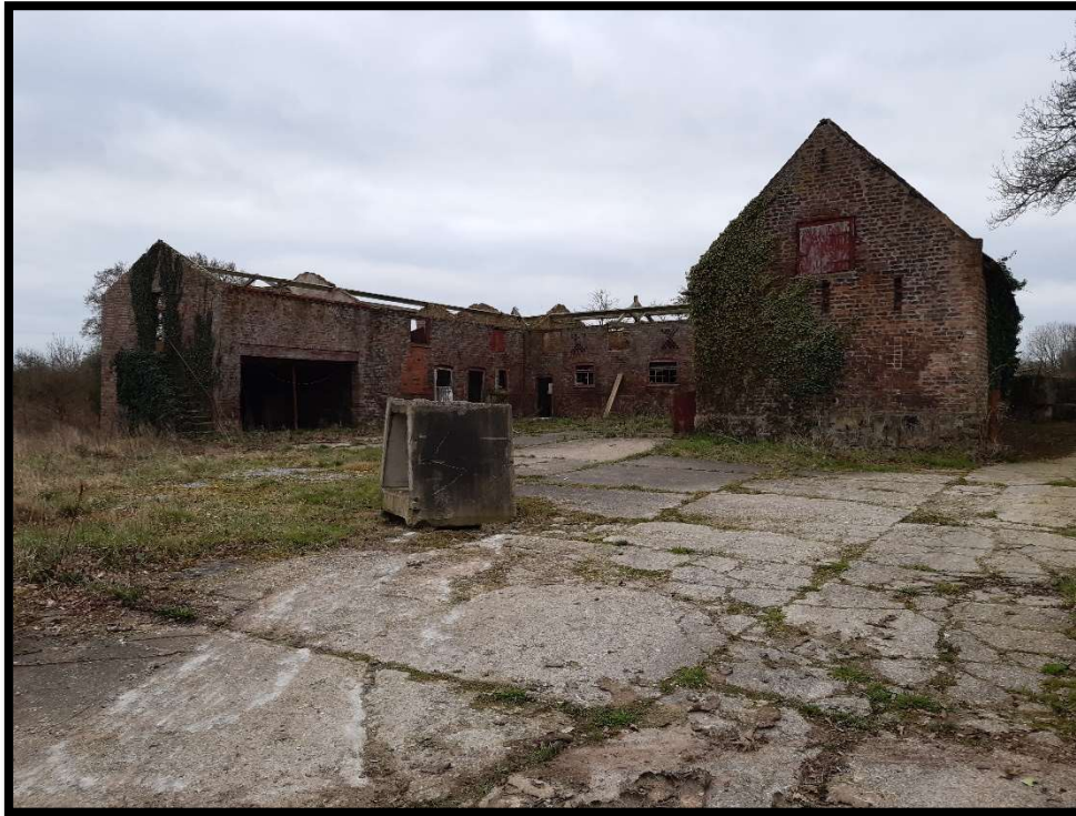
Photograph 1. Looking south at derelict farm buildings.
