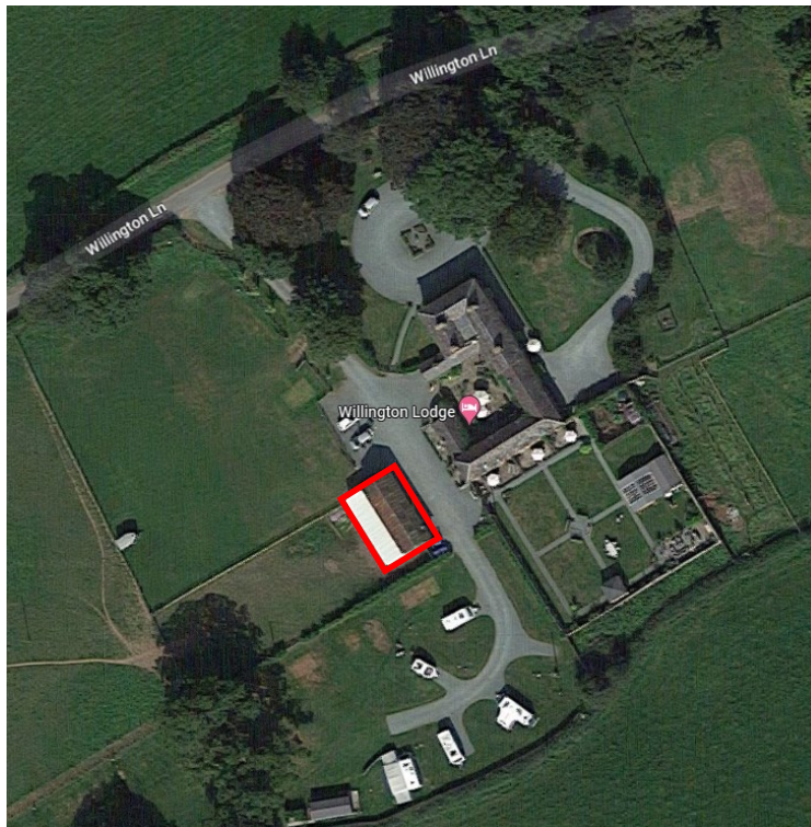
Aerial Image of Willington Lodge in Whitchurch
