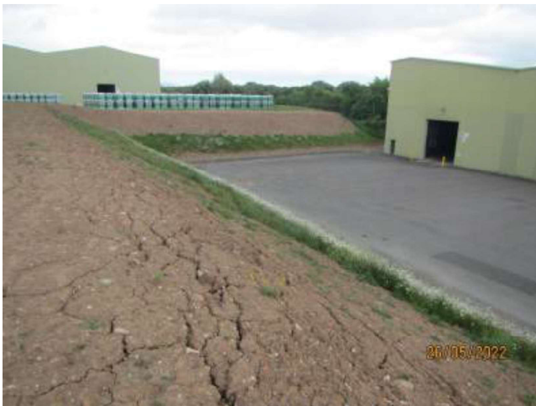
Photo 7. Looking eastwards from the north of the site boundary for Extension 2.
