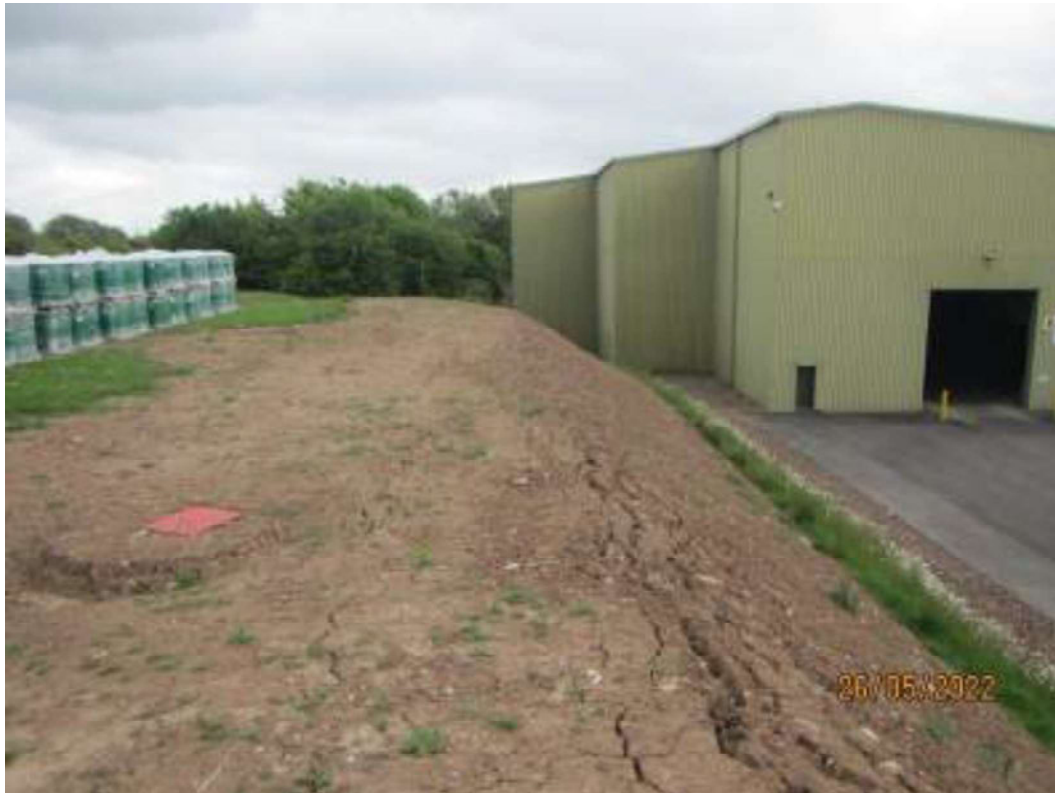
Photo 9. Looking south-east towards the building with Extension 2.
