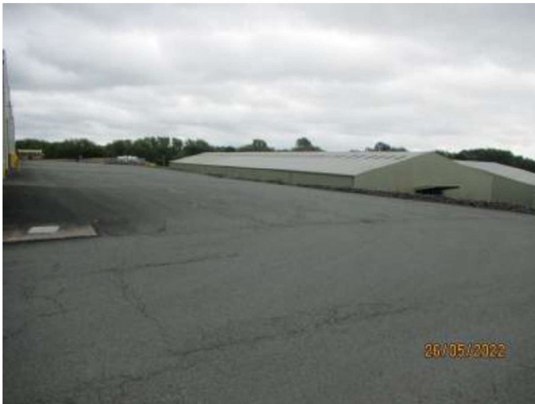
Photo 19. Example of roads running through the site.
