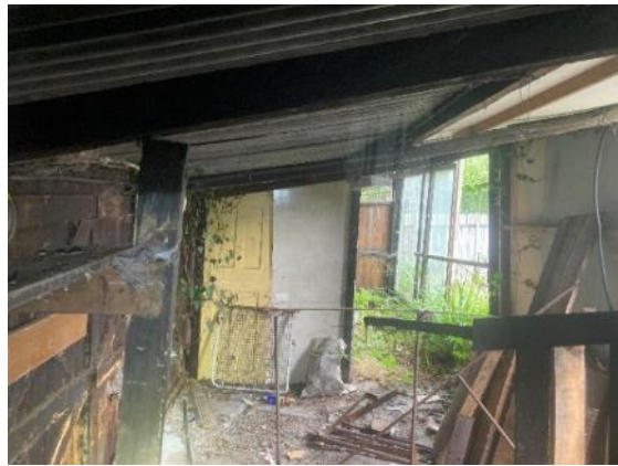
Plate 2. Building B3 internal
