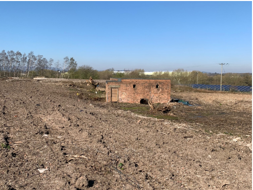
Paint store - Exterior Image prior to removal
