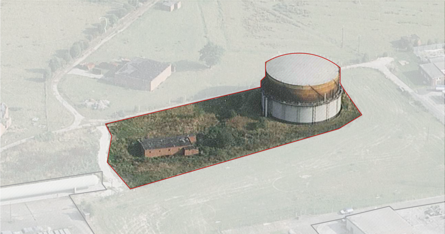
Gas holder and paint store - highlighted aerial image
