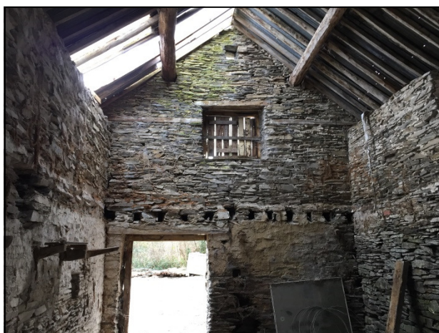
Plate 2 Looking south through barn
