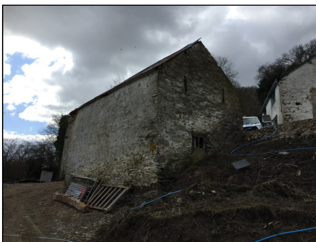
Plate 4 The external walls are well pointed
