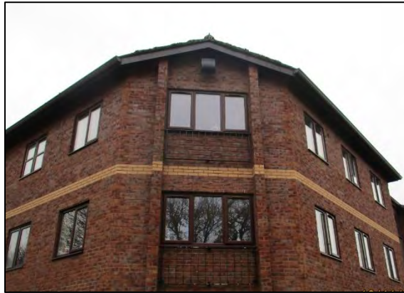
Figure 10: B01 showing soffit feature
