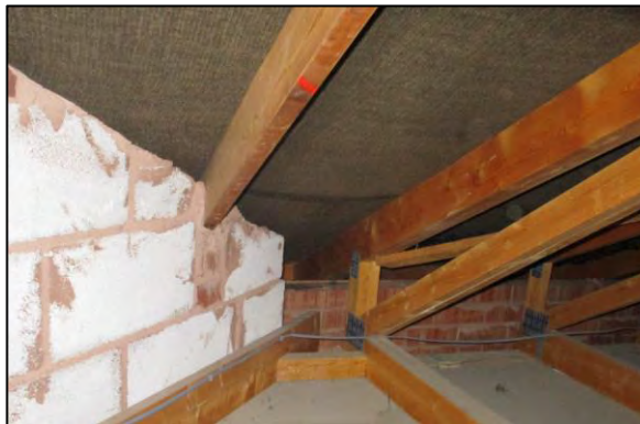
Figure 12: Internal roof structure of B01
