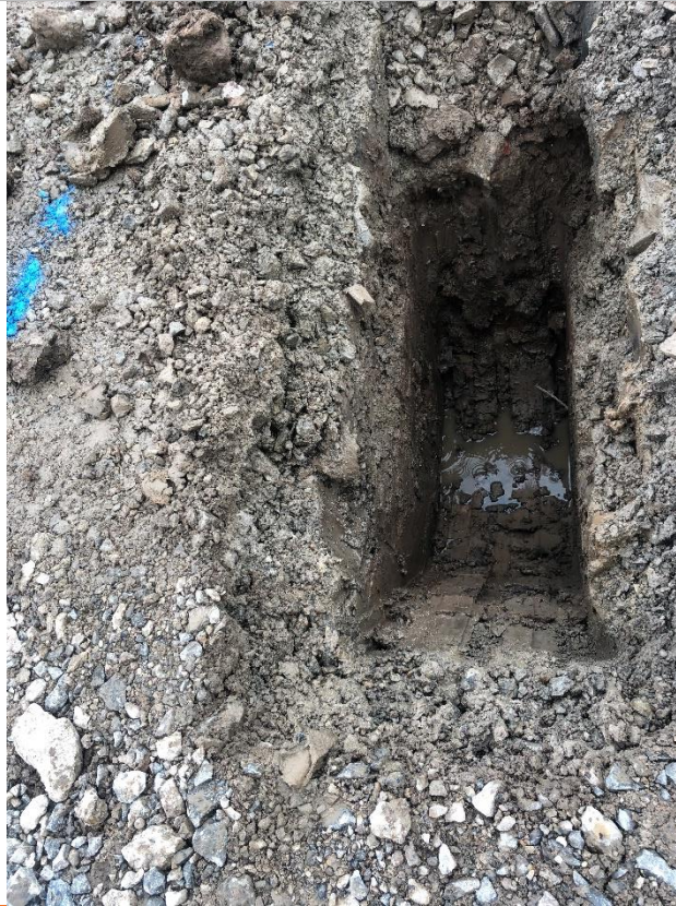
PLATE 1 SUPPLEMENTARY GROUND INVESTIGATION - TP201
