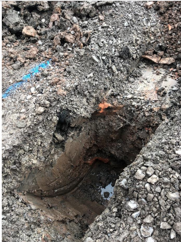
PLATE 2 SUPPLEMENTARY GROUND INVESTIGATION - TP203
