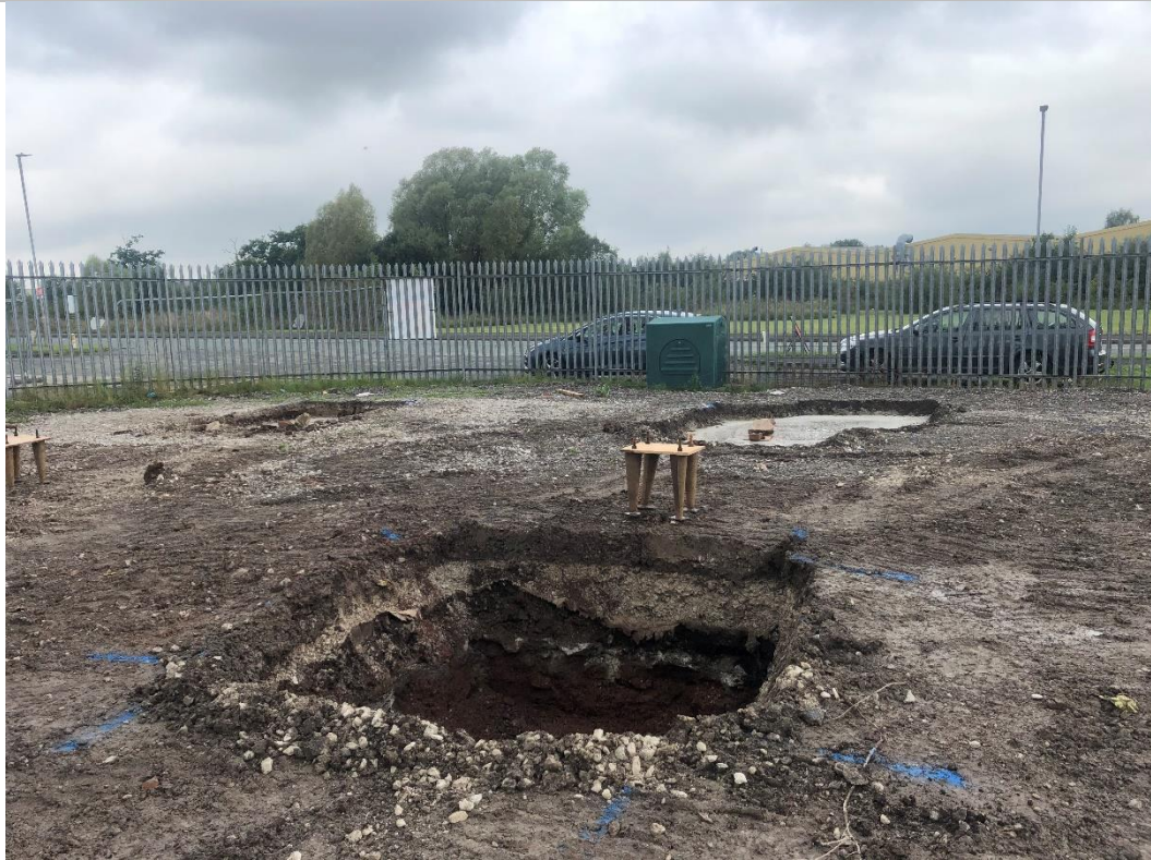
PLATE 3 PAD FOUNDATIONS INSTALLED ACROSS AREA OF HISTORIC POND
