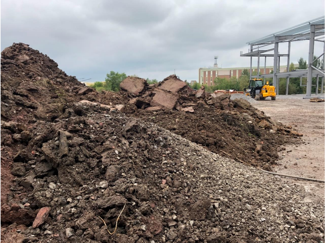
PLATE 7 STOCKPILE OF EXCESS MADE GROUND MATERIALS
