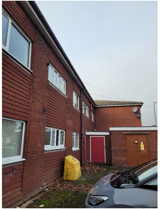
Photo 5 Soffit overhang and small flat-roofed extension in north
