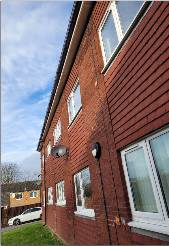
Photo 4 Example of the brickwork and decorative tiling
