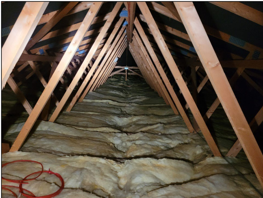
Photo 6 Example of the internal loft space
