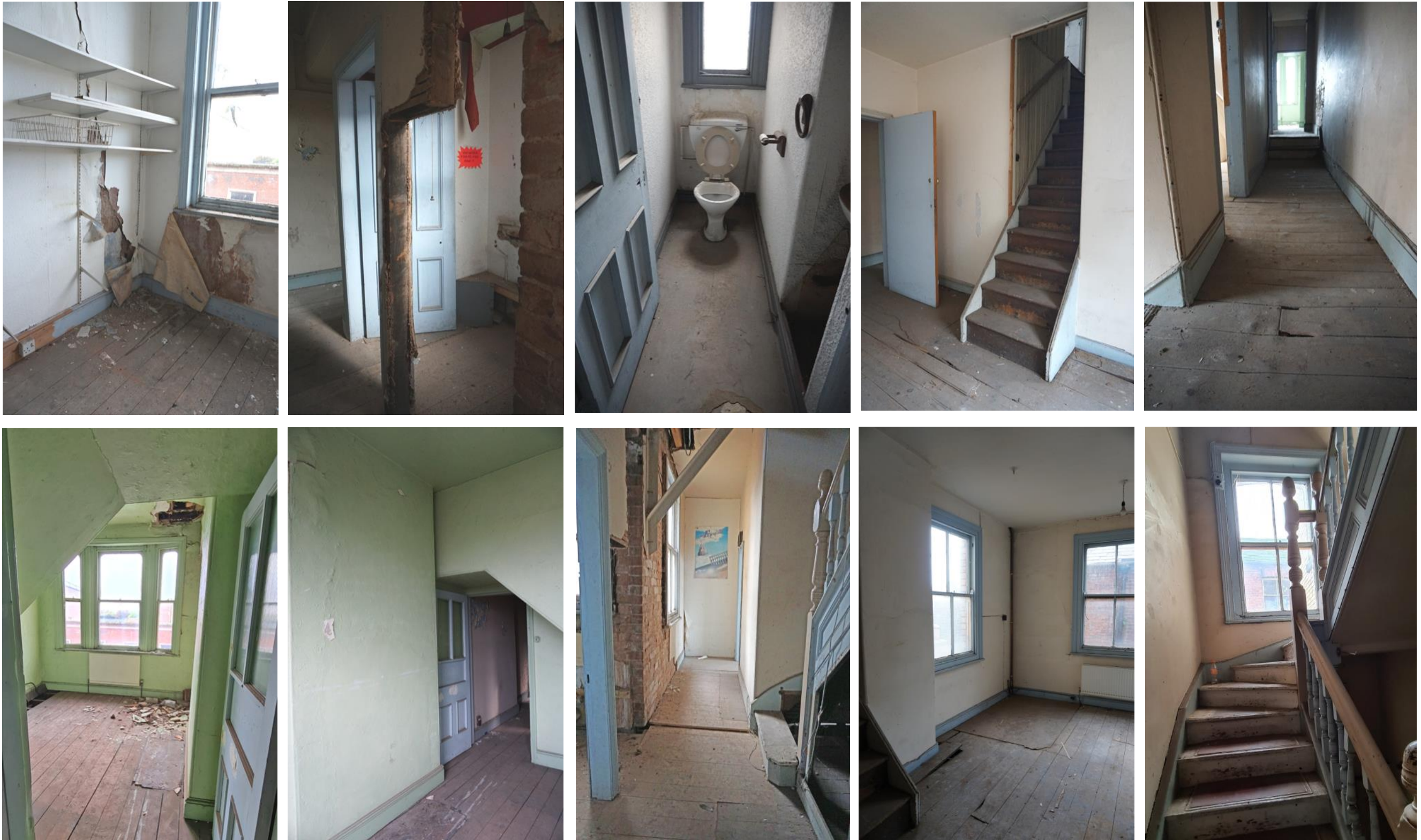
EXISTING SECOND FLOOR PHOTOGRAPHS
