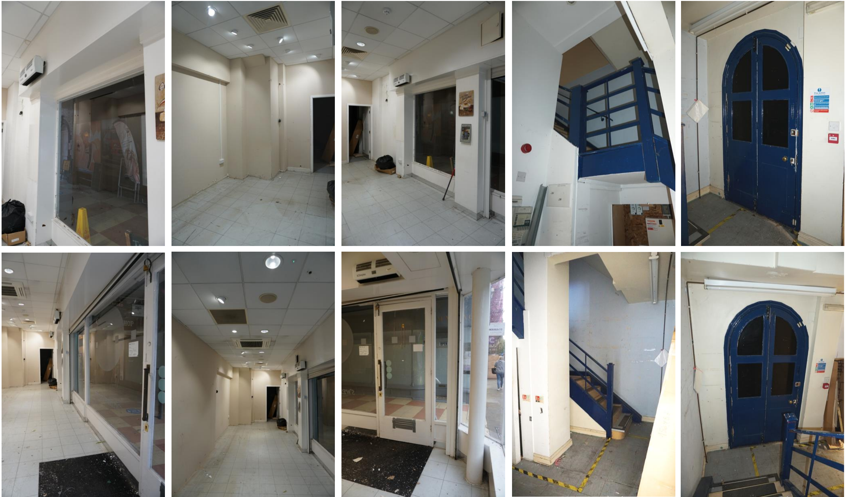
EXISTING GROUND FLOOR PHOTOGRAPHS
