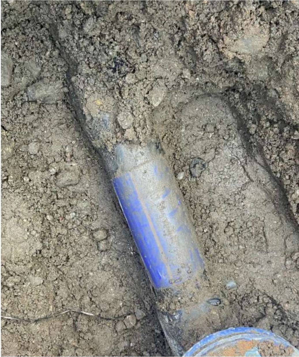
PE Pipe at Jacques Yard on Jacques Way in Wrexham
