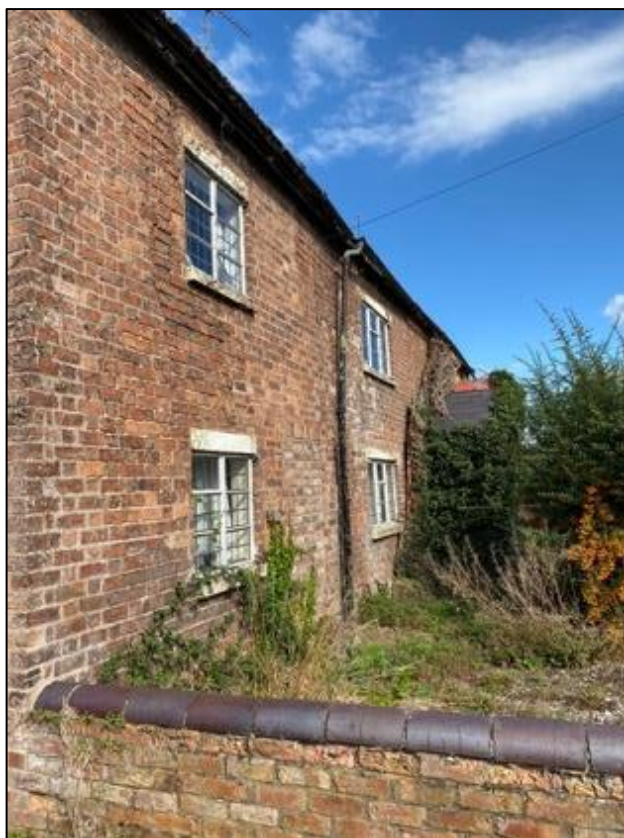
Fig 4: Showing the front elevation of the main target building.
