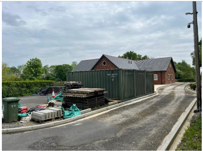
Southern edge of compound fitted with curbs.
