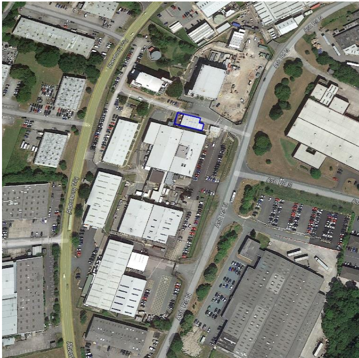
Fig 1 Aerial view of EAST site from 2018 prior to the demolition of Proserve
