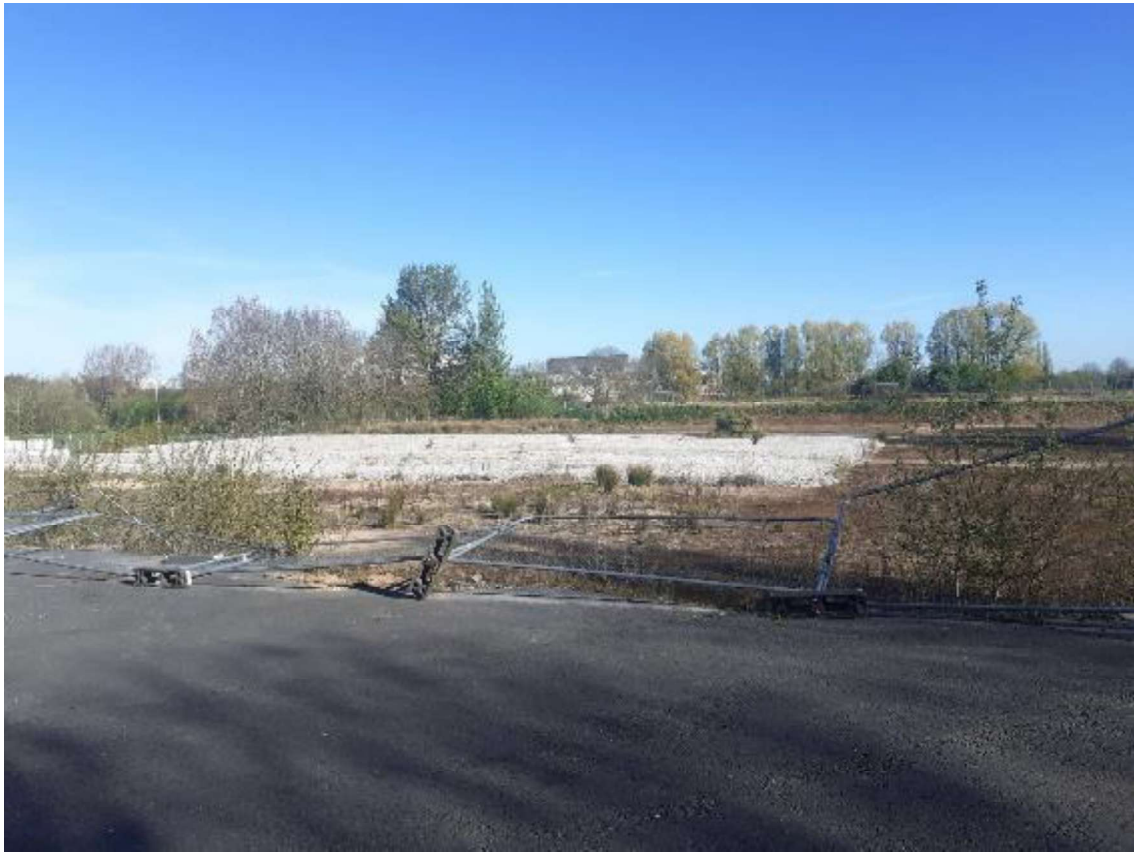
PLATE 5 VIEW OF THE SITE FACING NORTH
