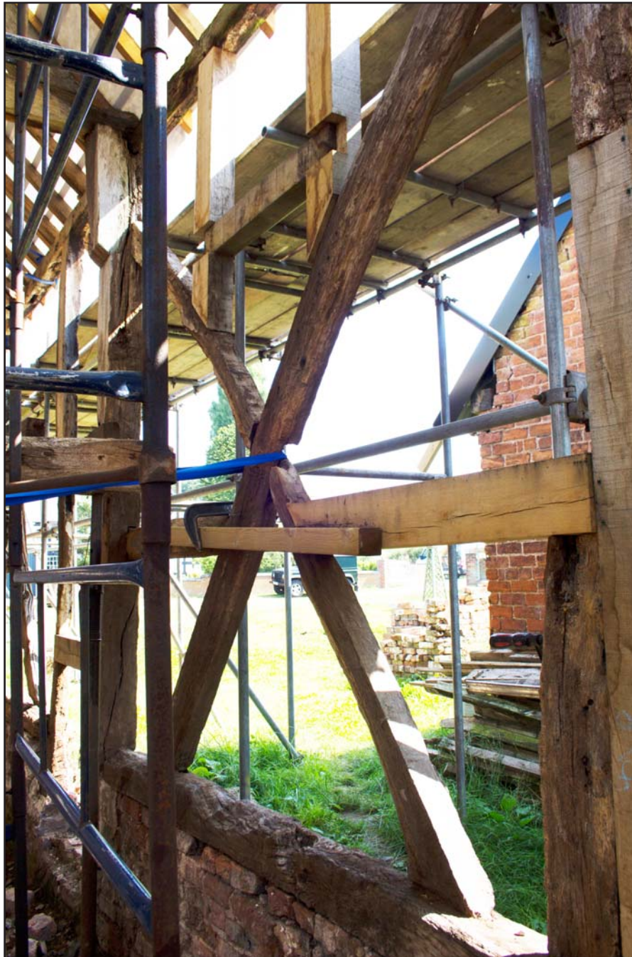
Plate 54: Full height diagonal cross braces in Room 6, ground floor, Shippon 1 at Brunette Farm, Ty Broughton, Wrexham - from the west - no scale
