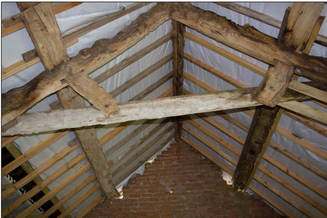
Plate 23: North western handhewn truss in Room 3, Stable at Brunette Farm, Ty Broughton, Wrexham - from the southeast - no scale
