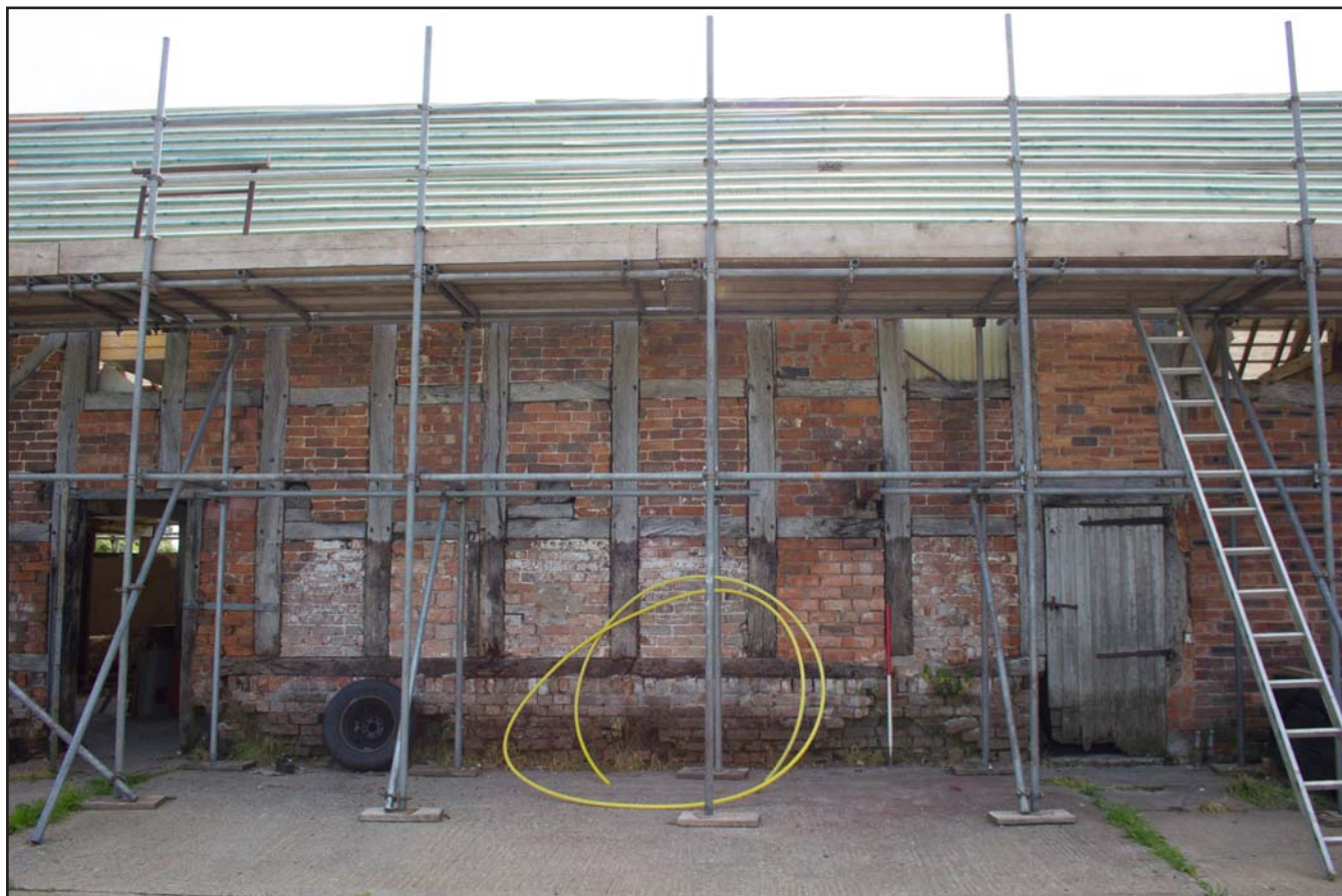
Plate 34: Centre of northwest elevation of Shippon 1 at Brunette Farm, Ty Broughton, Wrexham - from the northwest - scale 1m
