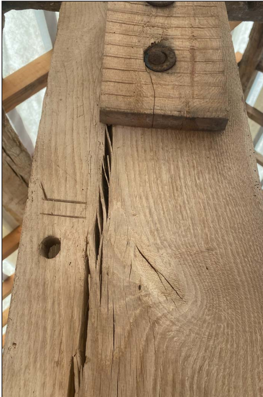
Plate 63: Carpenter's marks (II) on northwest stud, Truss 2 within Shippon 1 at Brunette Farm, Ty Broughton, Wrexham - from the southwest - no scale
