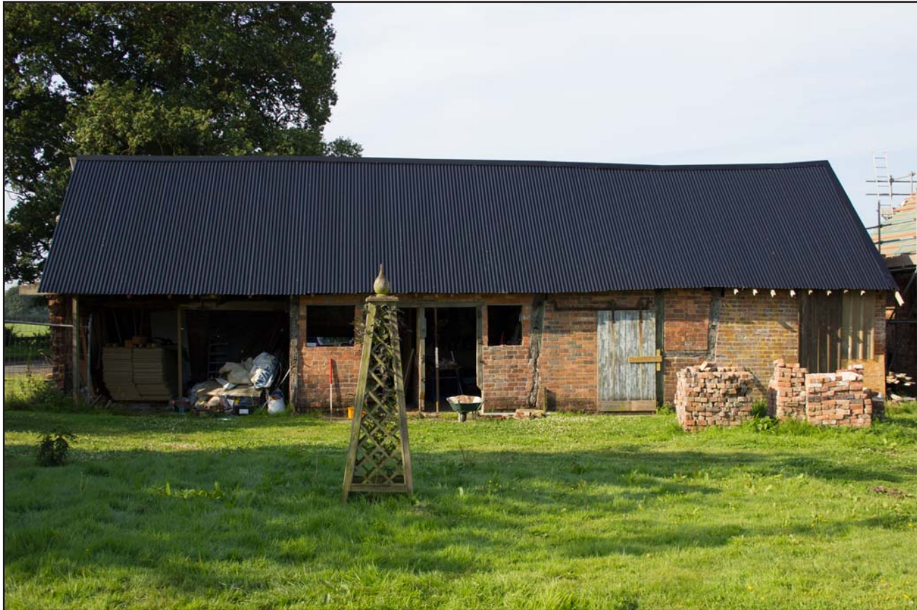
Plate 01: Northeast facing elevation of the Stable Building at Brunette Farm, Ty Broughton, Wrexham - from the northeast - scale 1m
