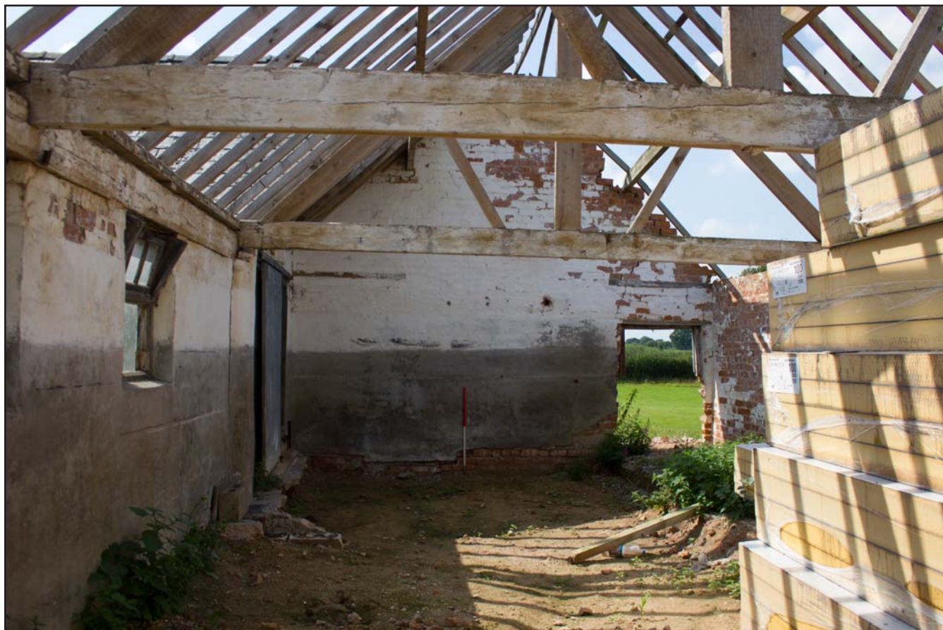
Plate 89: Internal shot of Shippon 3 at Brunette Farm, Ty Broughton, Wrexham - from the northeast - 1m scale
