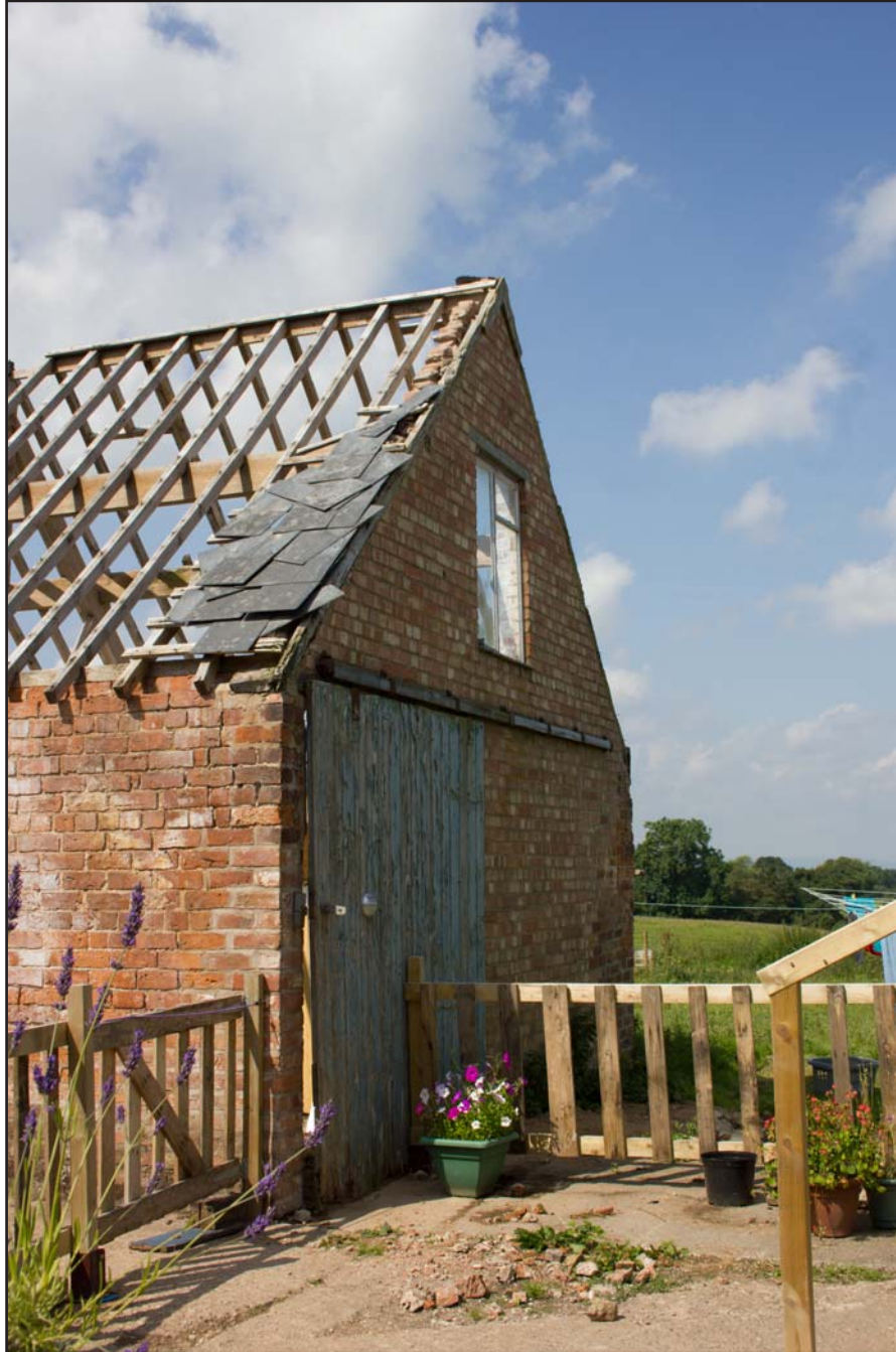
Plate 84: Northeast facing elevation of Shippon 3 at Brunette Farm, Ty Broughton, Wrexham - from the northeast - 1m scale
