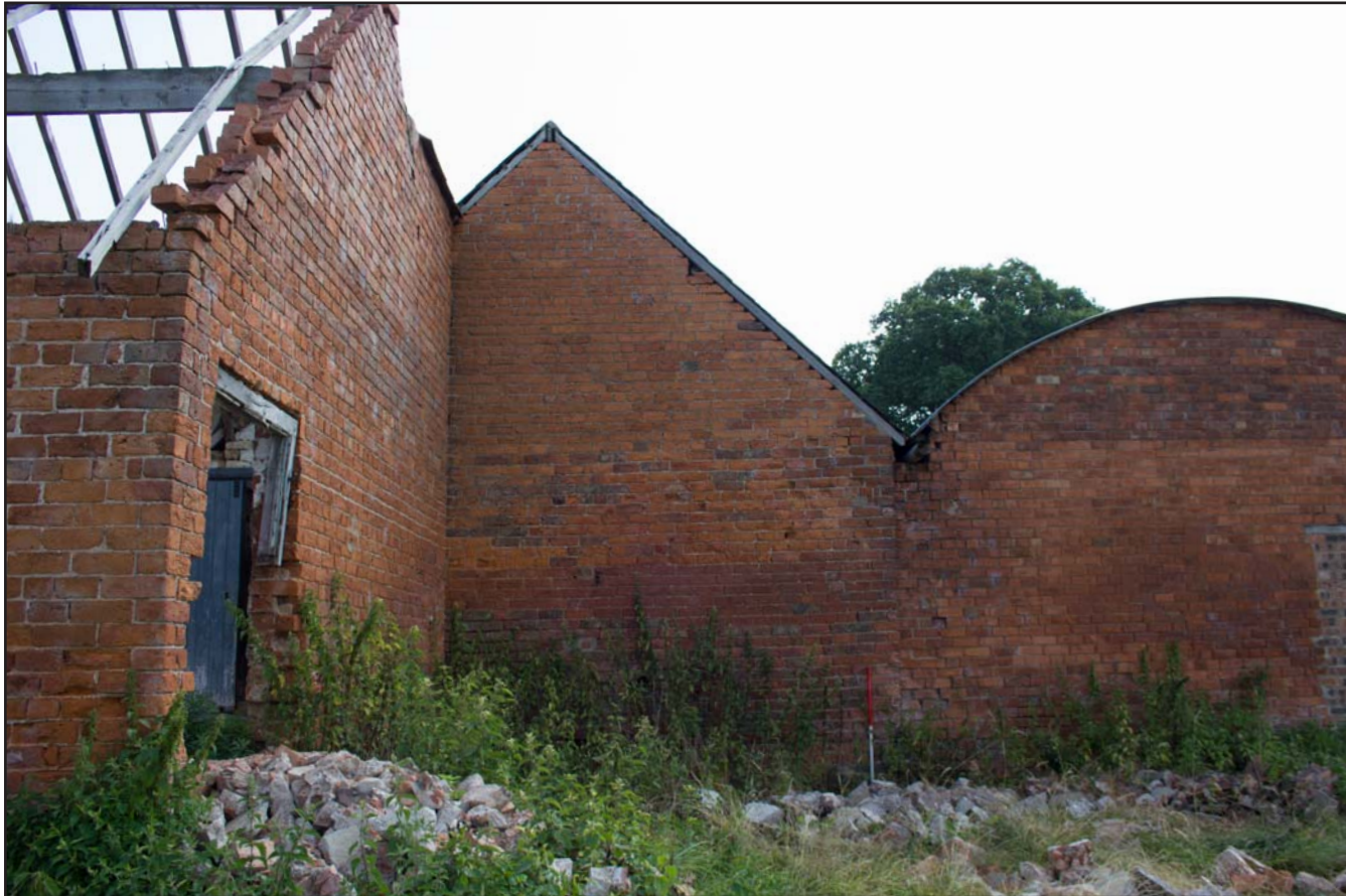
Plate 77: Northwest facing elevation of Shippon 2 at Brunette Farm, Ty Broughton, Wrexham - from the northwest - 1m scale
