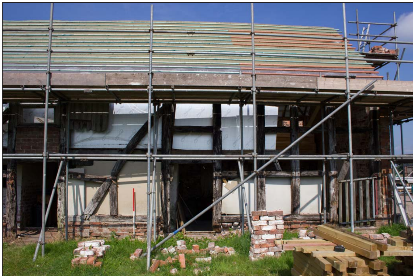
Plate 27: Far right hand end of southeast elevation of Shippon 1 at Brunette Farm, Ty Broughton, Wrexham - from the southeast - scale 1m
