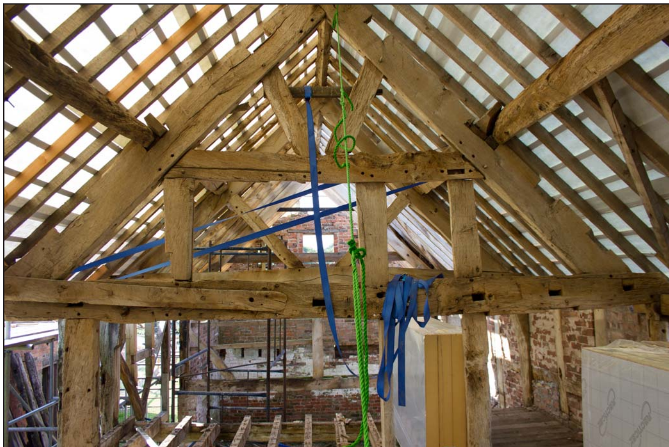
Plate 57: Truss 1, First floor, Shippon 1 at Brunette Farm, Ty Broughton, Wrexham - from the northeast - no scale
