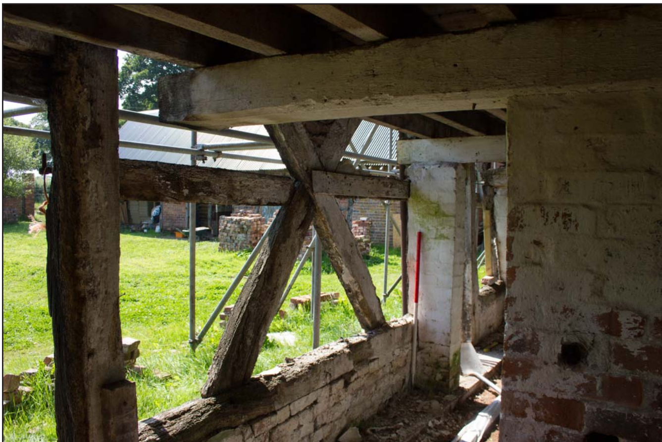
Plate 44: Full height diagonal cross braces in Room 1 and passageway, ground floor, Shippon 1 at Brunette Farm, Ty Broughton, Wrexham - from the north - no scale
