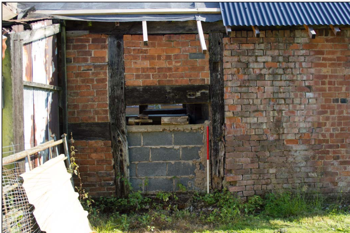
Plate 06: Right hand end of southwest elevation of the Stable at Brunette Farm, Ty Broughton, Wrexham - from the southwest - scale 1m
