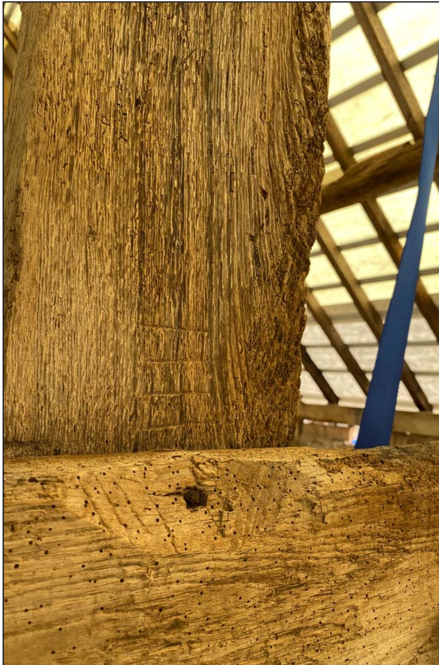
Plate 66: Carpenter's marks (III) on northwest stud, Truss 1 within Shippon 1 at Brunette Farm, Ty Broughton, Wrexham - from the southwest - no scale
