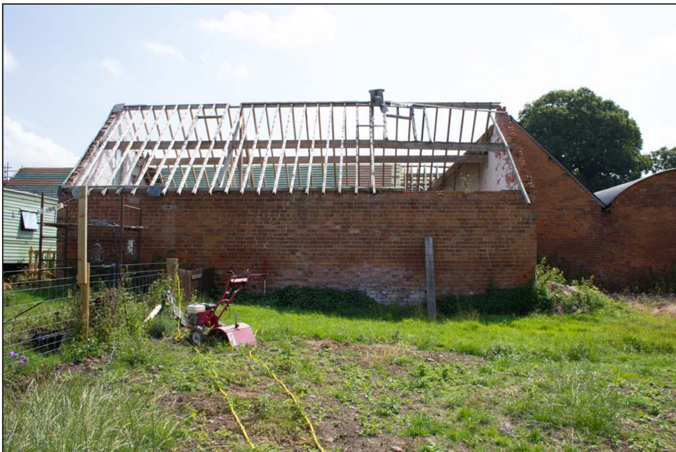
Plate 85: Northwest facing elevation of Shippon 3 at Brunette Farm, Ty Broughton, Wrexham - from the northwest - 1m scale
