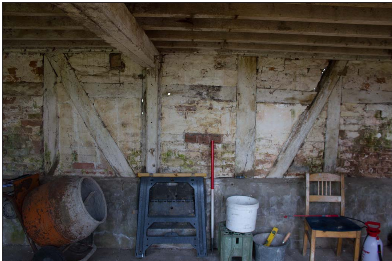
Plate 42: Northwest elevation within Room 1, ground floor, Shippon 1 at Brunette Farm, Ty Broughton, Wrexham - from the southeast - scale 1m
