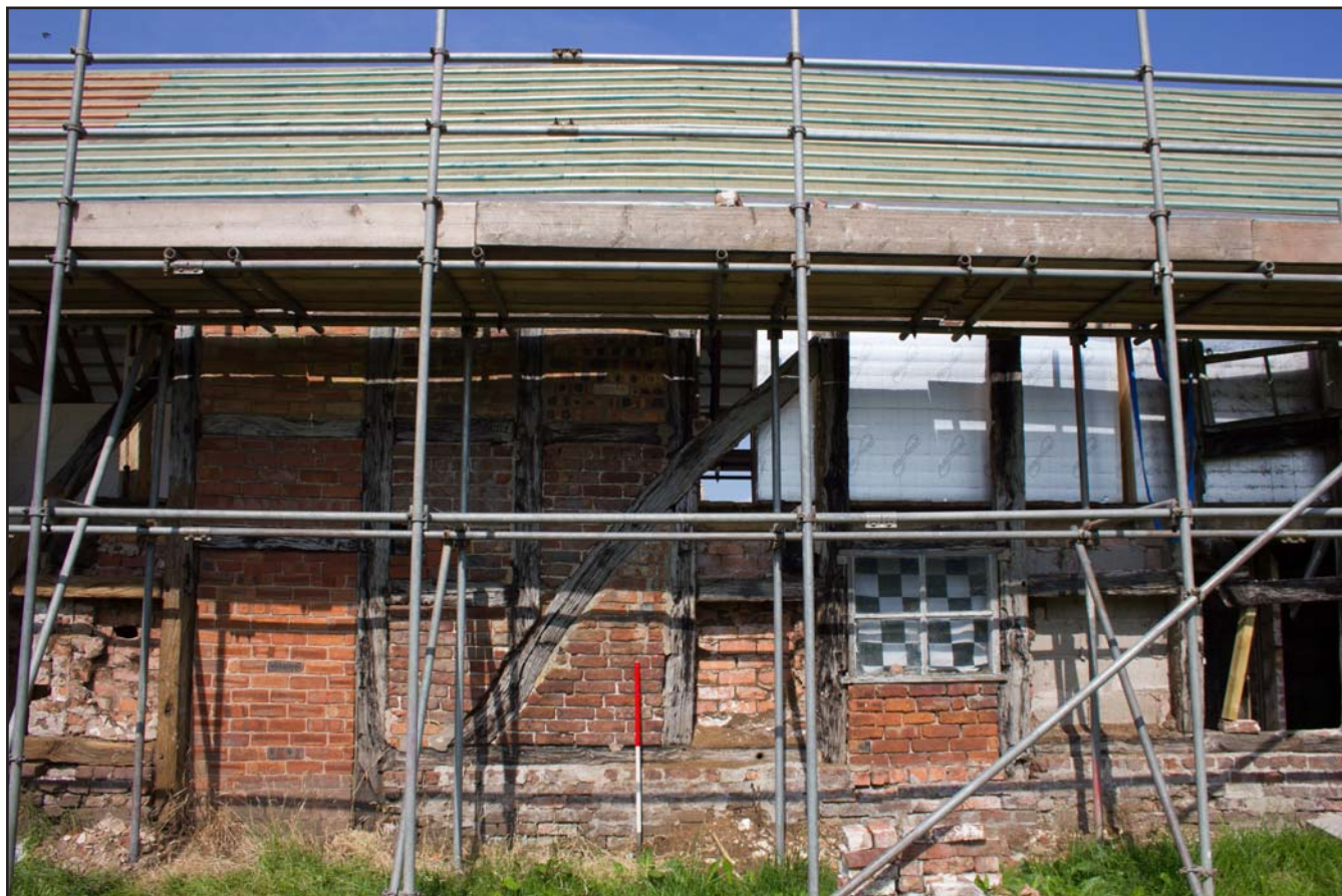
Plate 29: Far left hand end of southeast elevation of Shippon 1 at Brunette Farm, Ty Broughton, Wrexham - from the southeast - scale 1m
