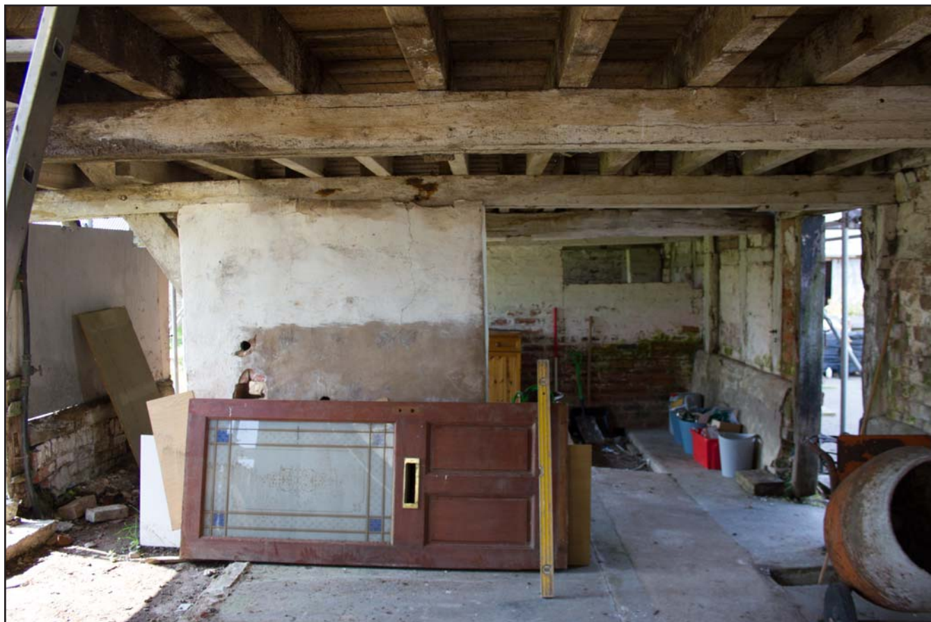
Plate 40: Room 1, ground floor within Shippon 1 at Brunette Farm, Ty Broughton, Wrexham - from the northeast - scale 1m
