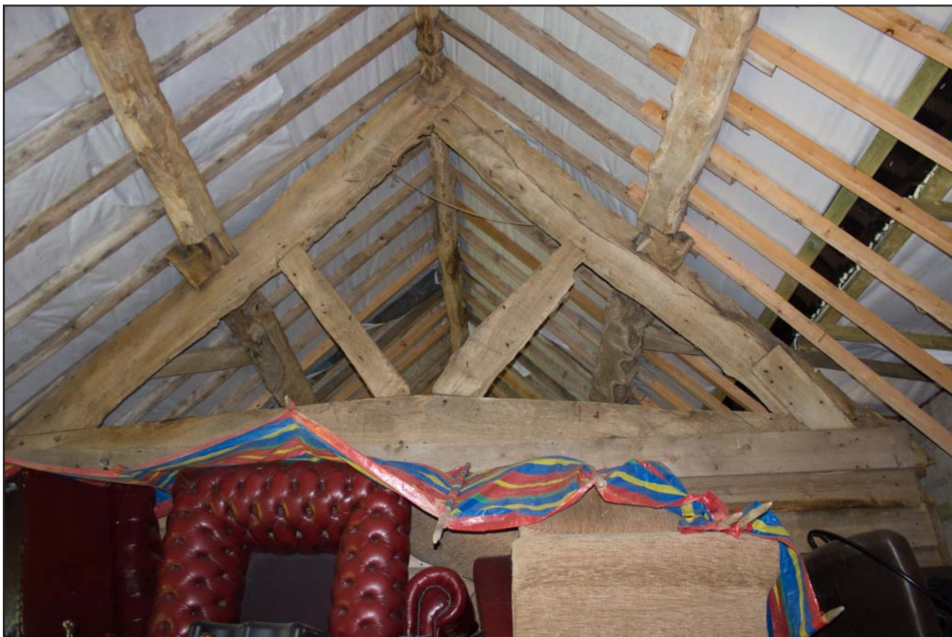
Plate 22: South eastern handhewn truss in Room 3, Stable at Brunette Farm, Ty Broughton, Wrexham - from the northwest - no scale
