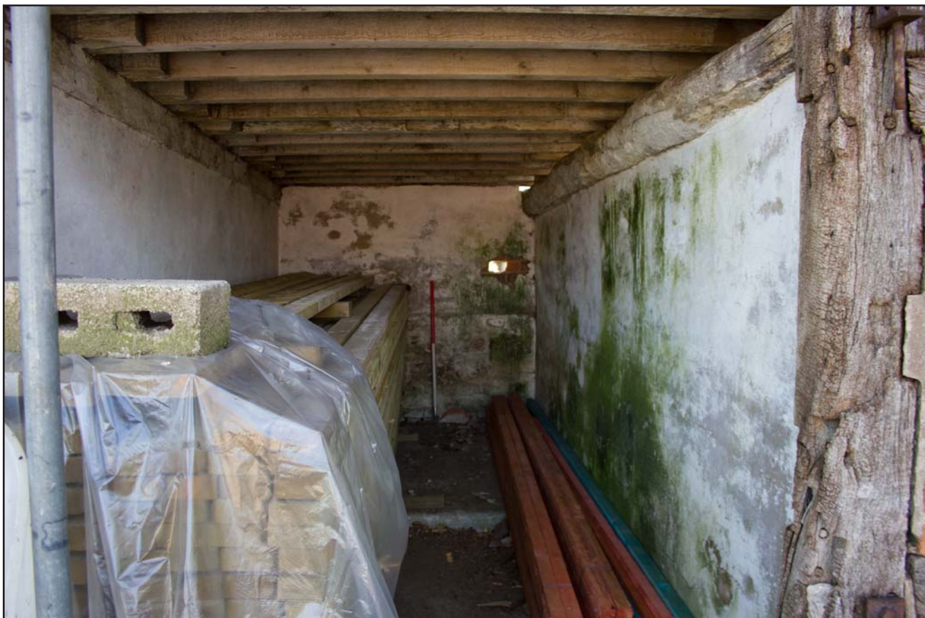
Plate 50: Room 5, ground floor, Shippon 1 at Brunette Farm, Ty Broughton, Wrexham - from the northwest - scale 1m
