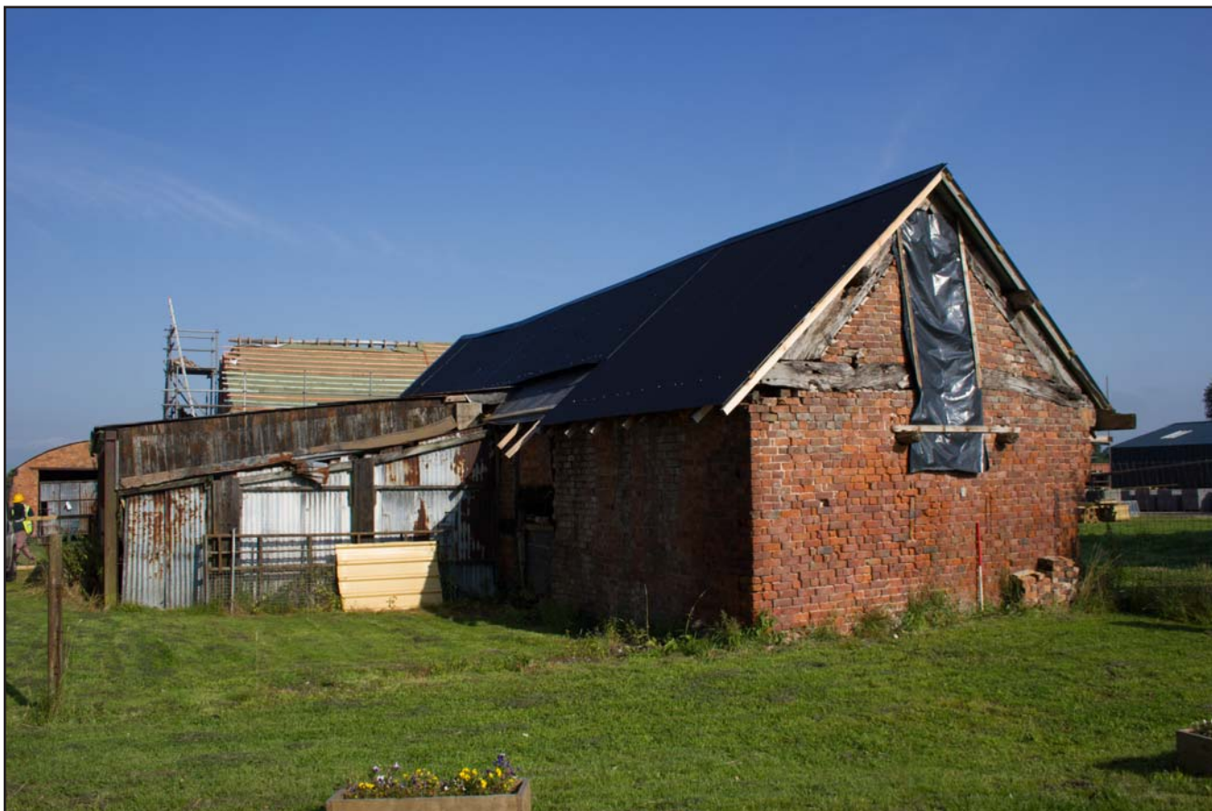
Plate 04: Southeast and southwest elevations of the Stable at Brunette Farm, Ty Broughton, Wrexham - from the south - scale 1m
