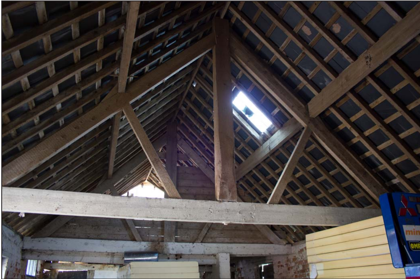
Plate 81: Kingspost truss within Shippon 2 at Brunette Farm, Ty Broughton, Wrexham - from the northwest - no scale
