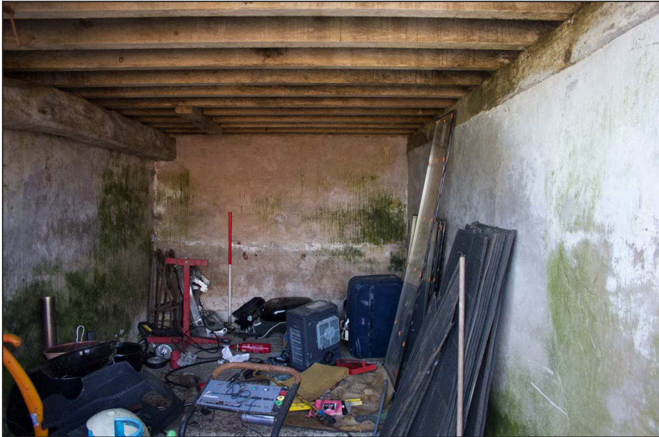
Plate 48: Room 4, ground floor, Shippon 1 at Brunette Farm, Ty Broughton, Wrexham - from the northwest - scale 1m
