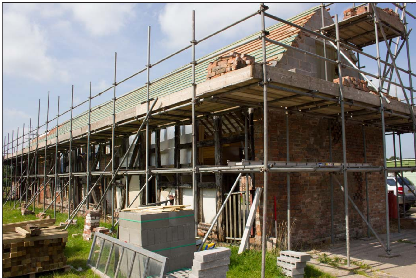
Plate 39: Northeast and northwest elevations of Shippon 1 at Brunette Farm, Ty Broughton, Wrexham - from the east - scale 1m
