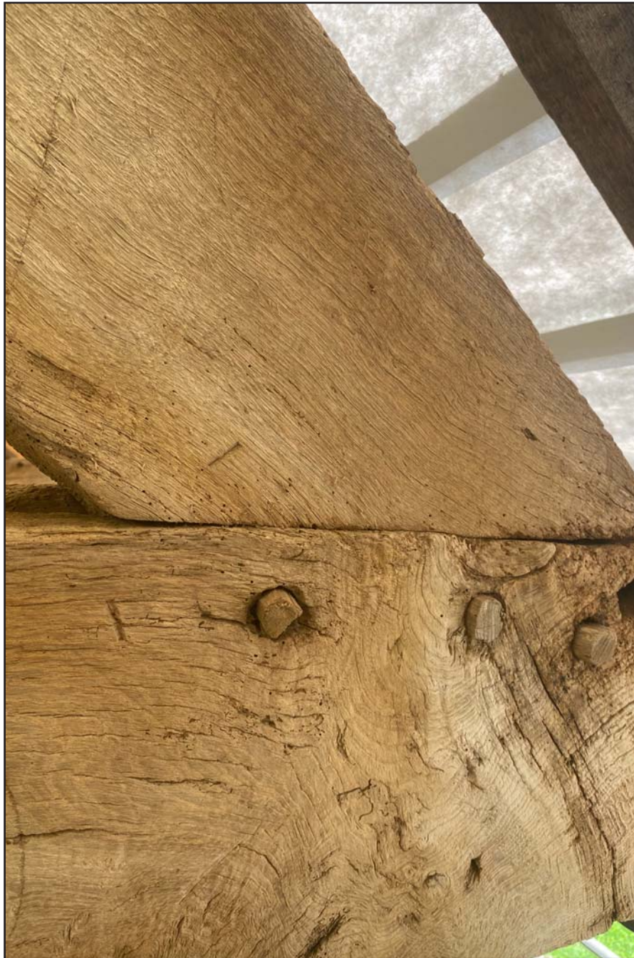
Plate 65: Carpenter's marks (II) on northwest rafter/tie-beam, Truss 3 within Shippon 1 at Brunette Farm, Ty Broughton, Wrexham - from the southwest - no scale
