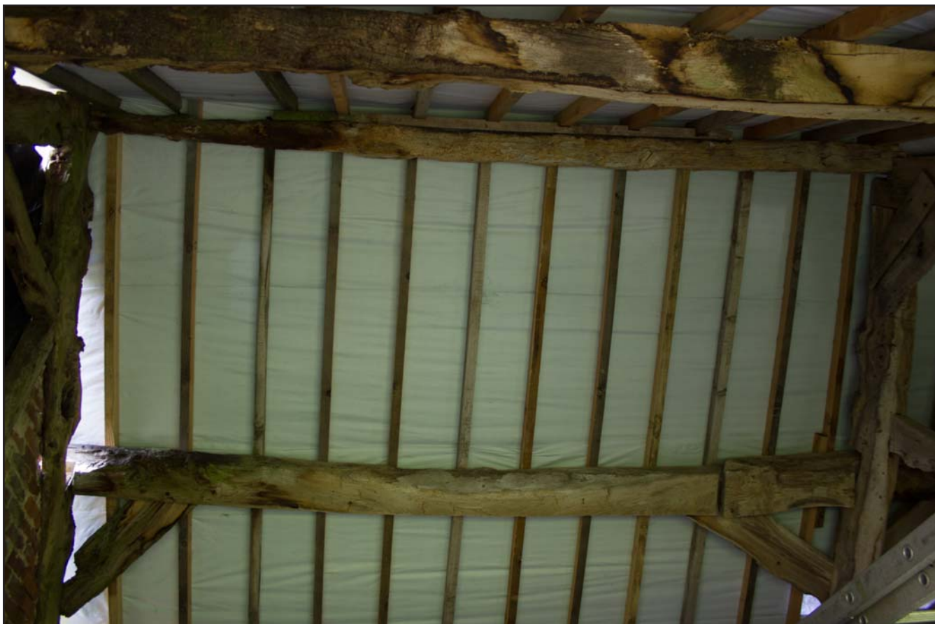
Plate 15: Handhewn purlins, ridgebeam and blade in Room 1, Stable at Brunette Farm, Ty Broughton, Wrexham - from the northeast - no scale
