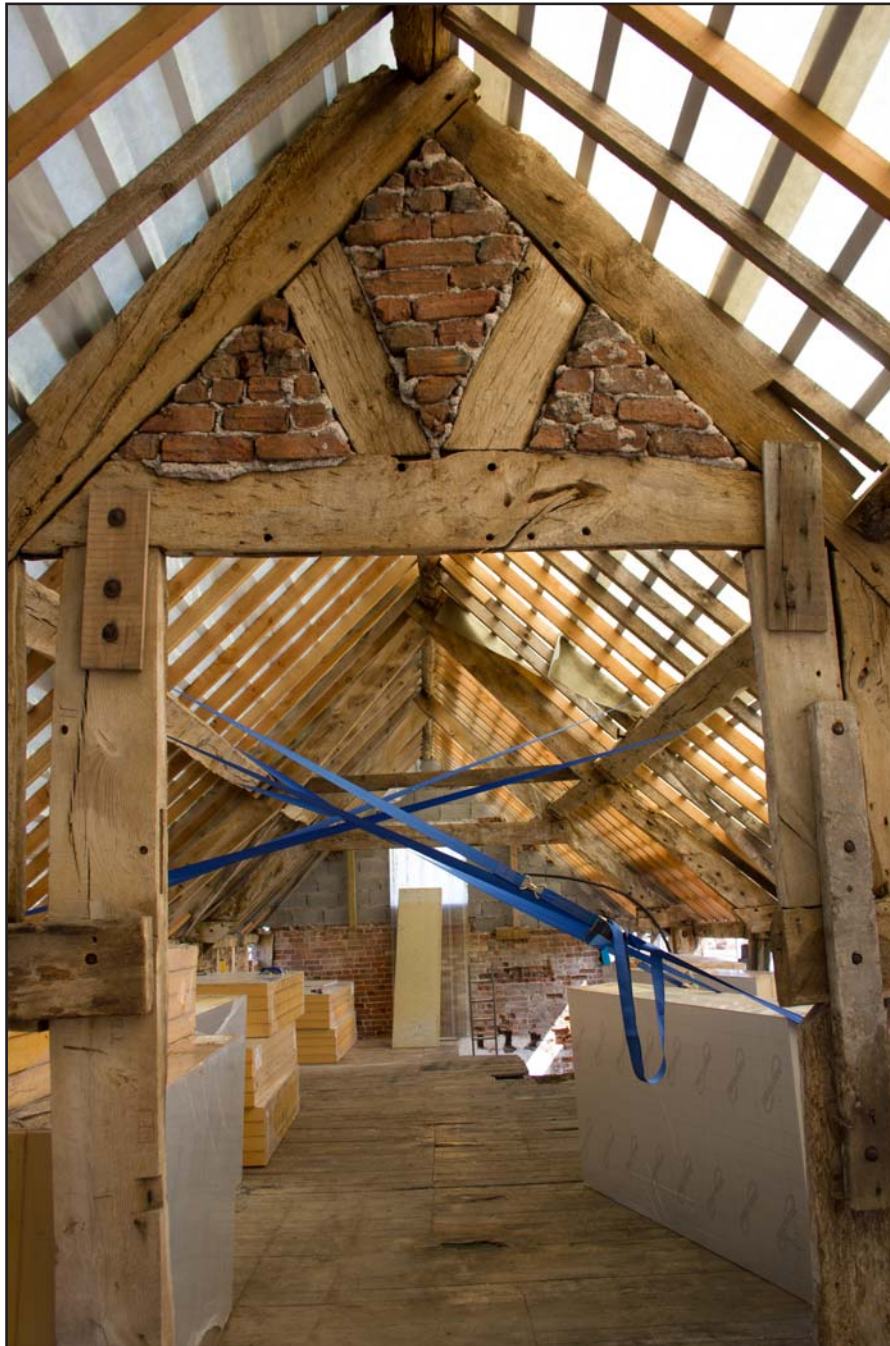
Plate 60: Crown/ridge of Truss 3, First floor, Shippon 1 at Brunette Farm, Ty Broughton, Wrexham - from the southwest - no scale
