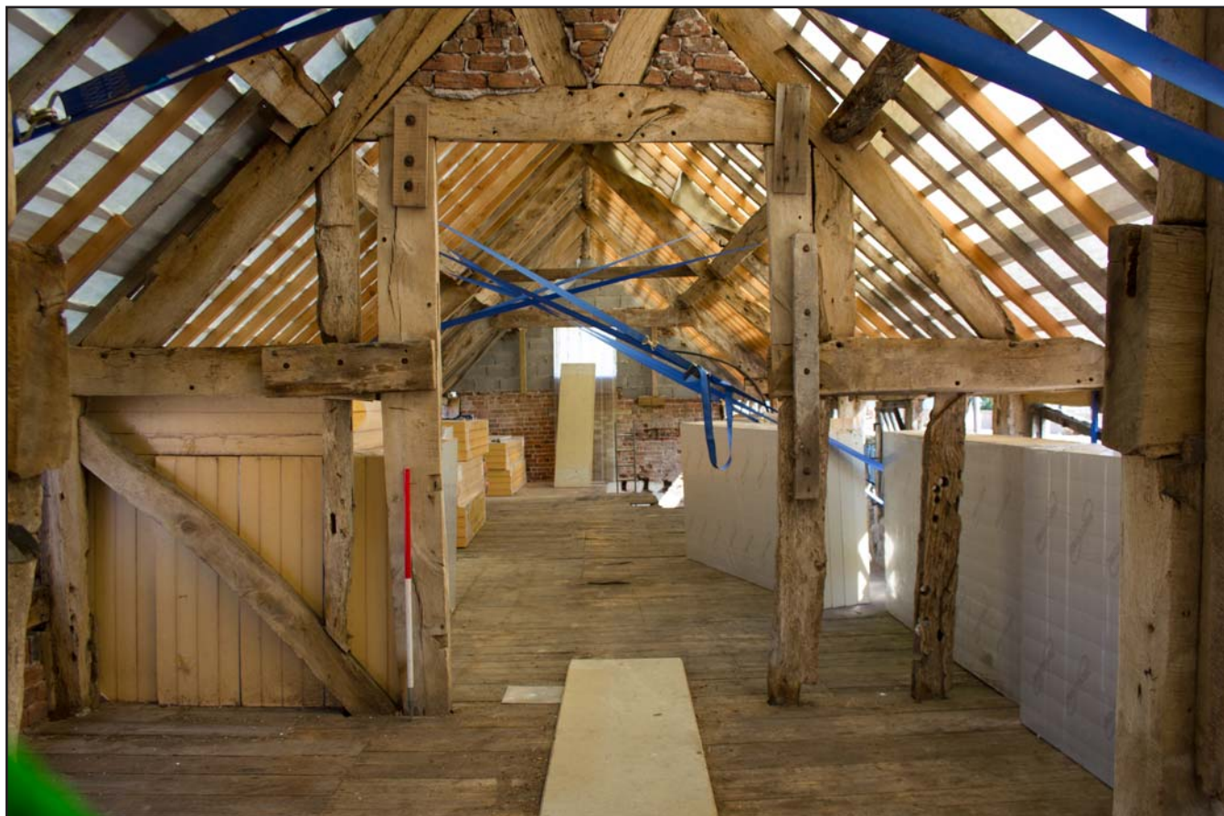
Plate 59: Truss 3, First floor, Shippon 1 at Brunette Farm, Ty Broughton, Wrexham - from the southwest - scale 1m
