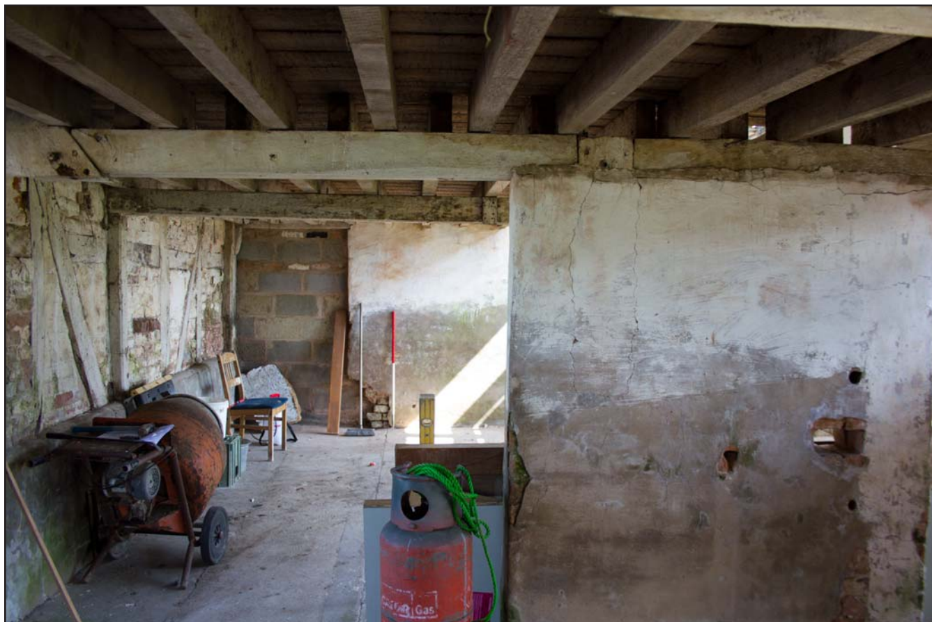
Plate 41: Room 1 , ground floor within Shippon 1 at Brunette Farm, Ty Broughton, Wrexham - from the southwest - scale 1m
