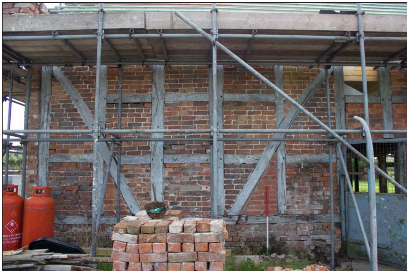
Plate 35: Left hand end of northwest elevation of Shippon 1 at Brunette Farm, Ty Broughton, Wrexham - from the north - scale 1m
