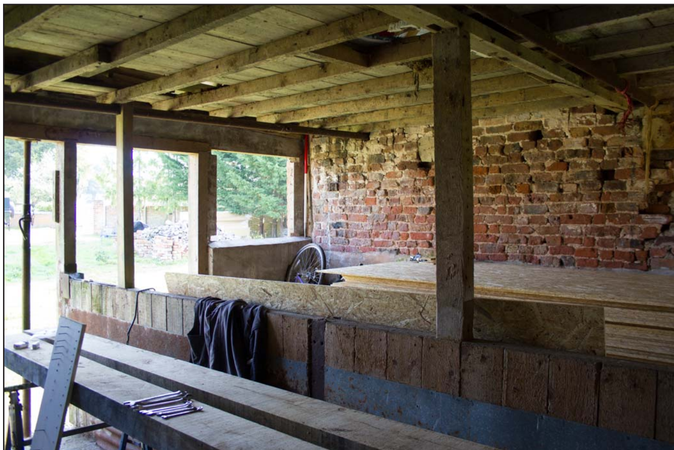
Plate 17: Room 2 within the Stable at Brunette Farm, Ty Broughton, Wrexham - from the west - scale 1m
