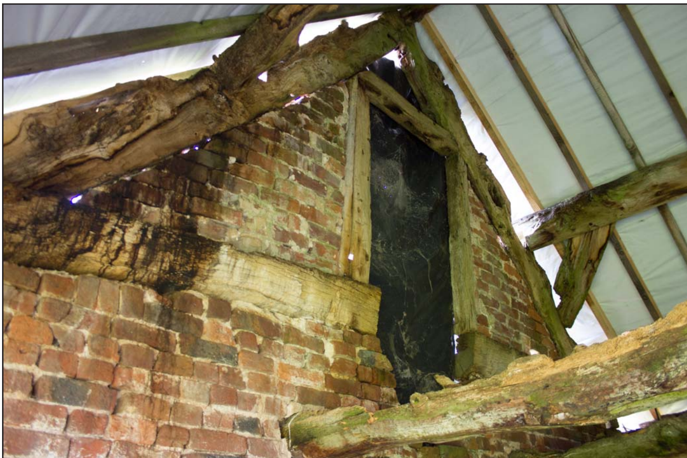
Plate 13: South eastern handhewn truss in Room 1, Stable at Brunette Farm, Ty Broughton, Wrexham - from the north - no scale
