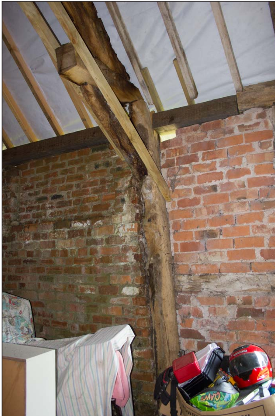
Plate 24: Handhewn upright post supporting north eastern trusse in Room 3, Stable at Brunette Farm, Ty Broughton, Wrexham - from the south - no scale
