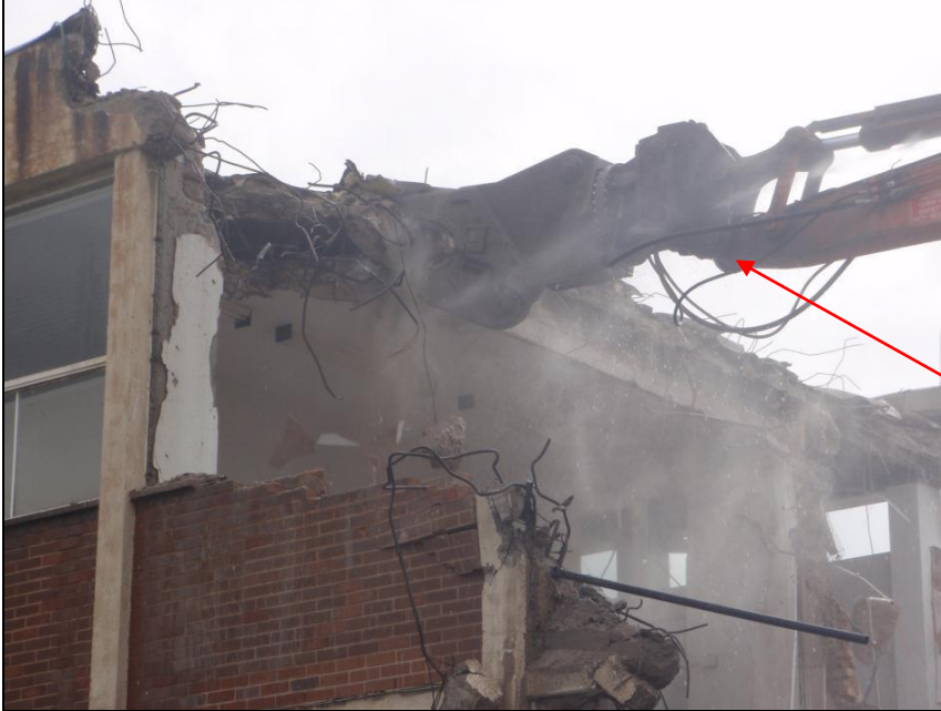
Dust suppression at source
