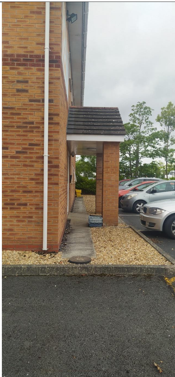
Photo 4 – from the north-eastern corner looking west, showing bare ground (gravel and slabs)
