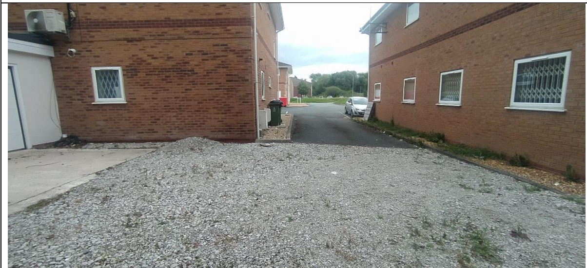
Photo 2 – from the south-eastern corner looking north, showing the building (extension to the left), bare ground (gravel and concrete)
