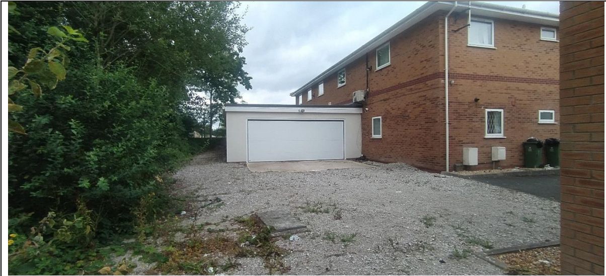
Photo 1 – from beyond the south-eastern corner looking west, showing the building (extension to the left), bare ground (gravel) and adjacent bramble scrub and broadleaved semi-natural woodland
