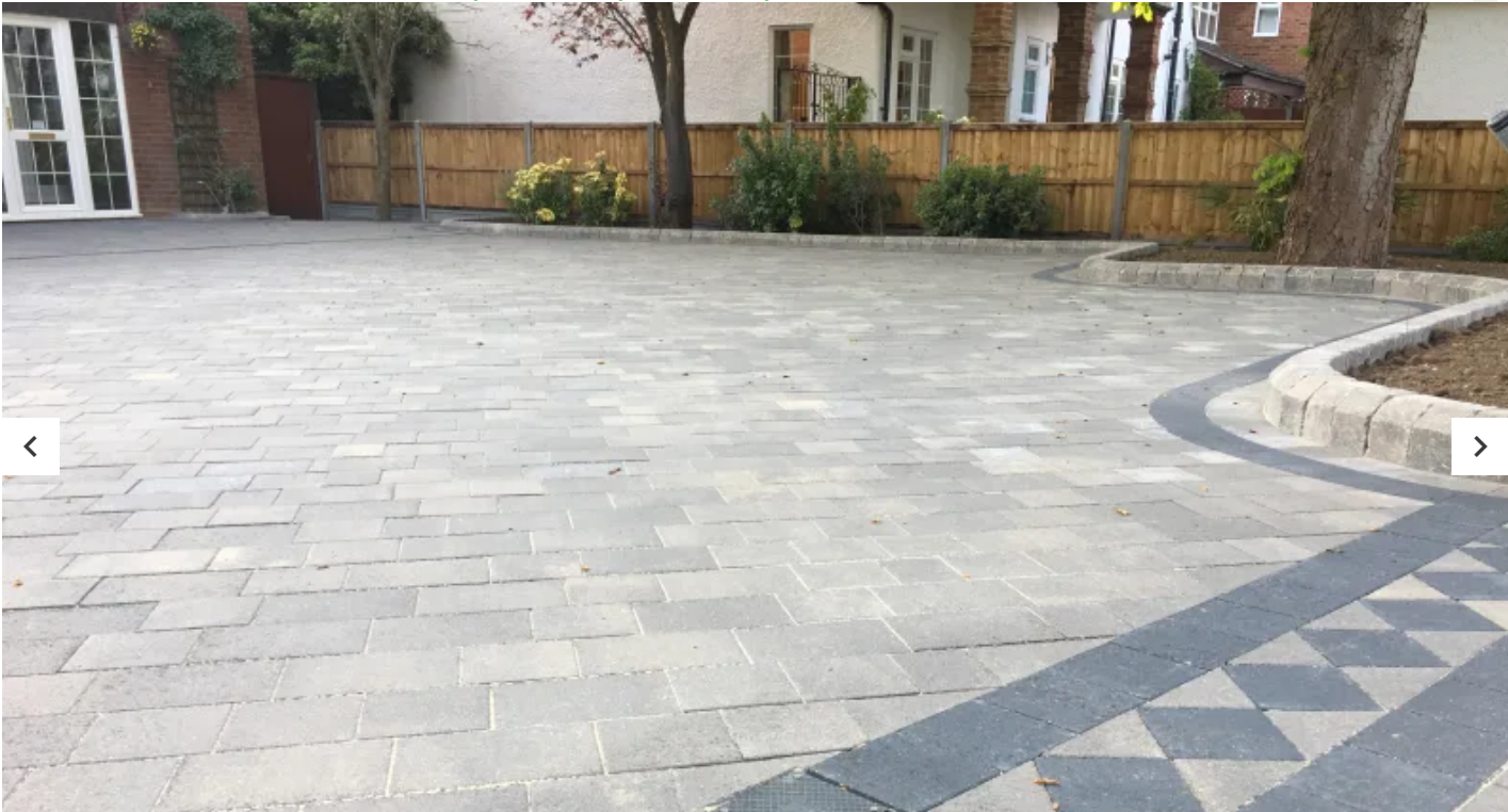
Marshalls Drivesett Savanna block paving in Grey
