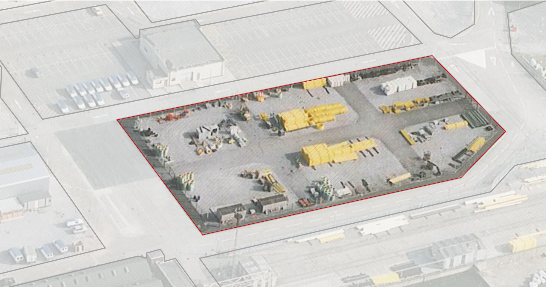
Open storage - highlighted aerial image
