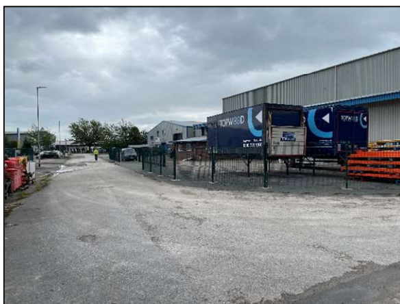
Figure 2: Looking southeast across the site.
