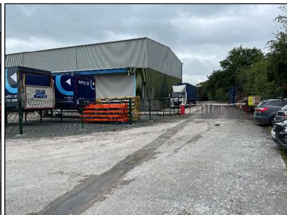
Figure 6: Looking south across the surveyed area.
