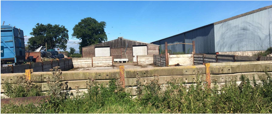
The existing slurry store to be covered.
