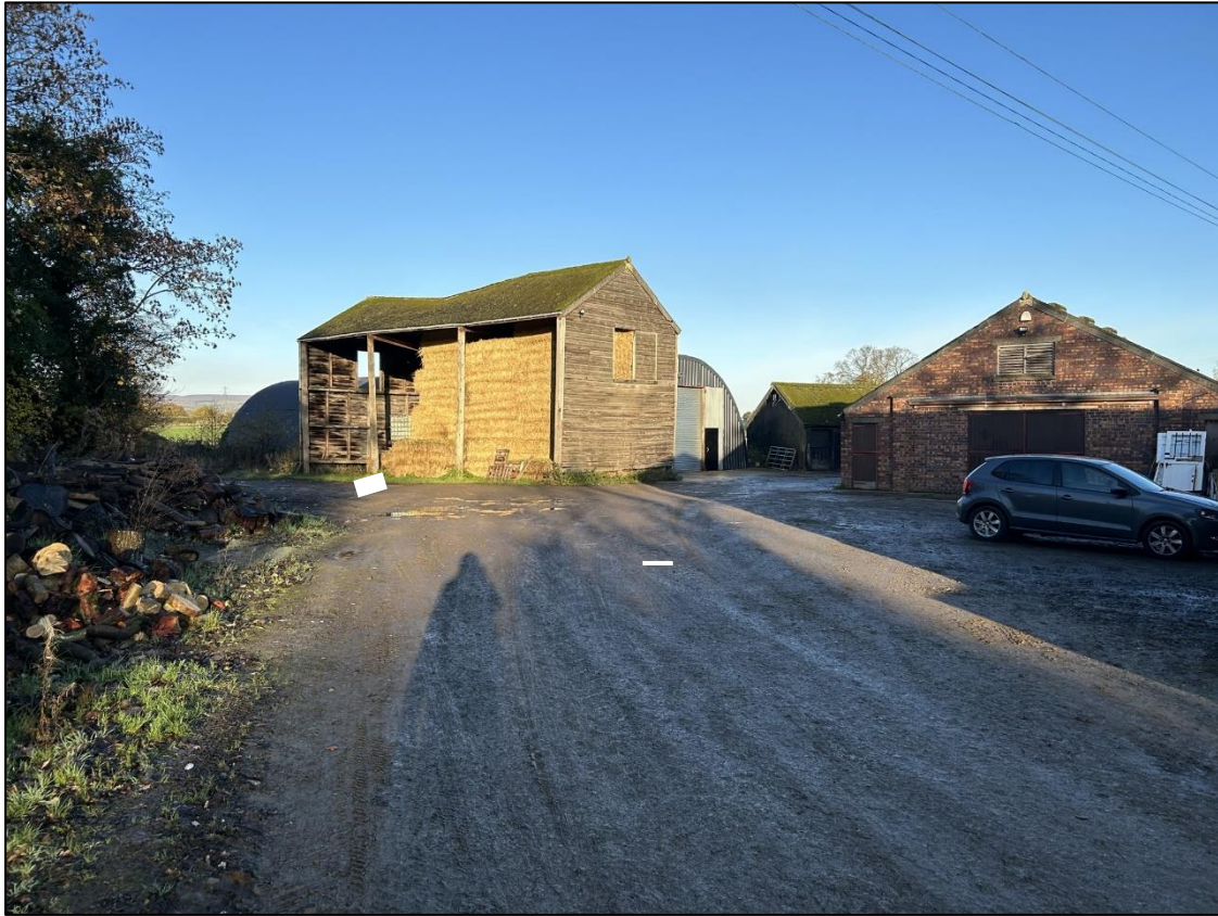
Plate 1 – Building B1 (right hand side) and building B3 (left hand side)
