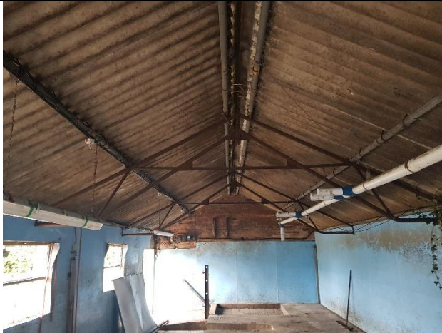
Internal conditions of the building.
