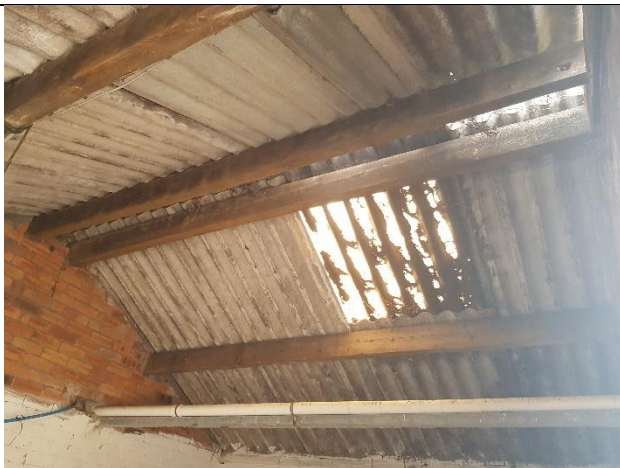
Sky lights in roof of building.
