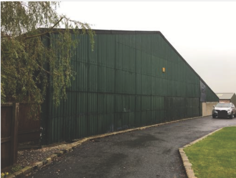
PHOTO 3: West Elevation of former portal-framed building (now removed by applicant)
