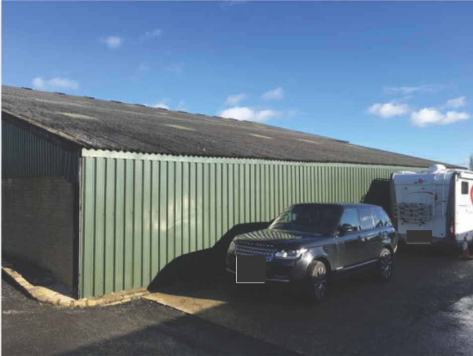
PHOTO 2: South Elevation of former portal-framed building (now removed by applicant)
