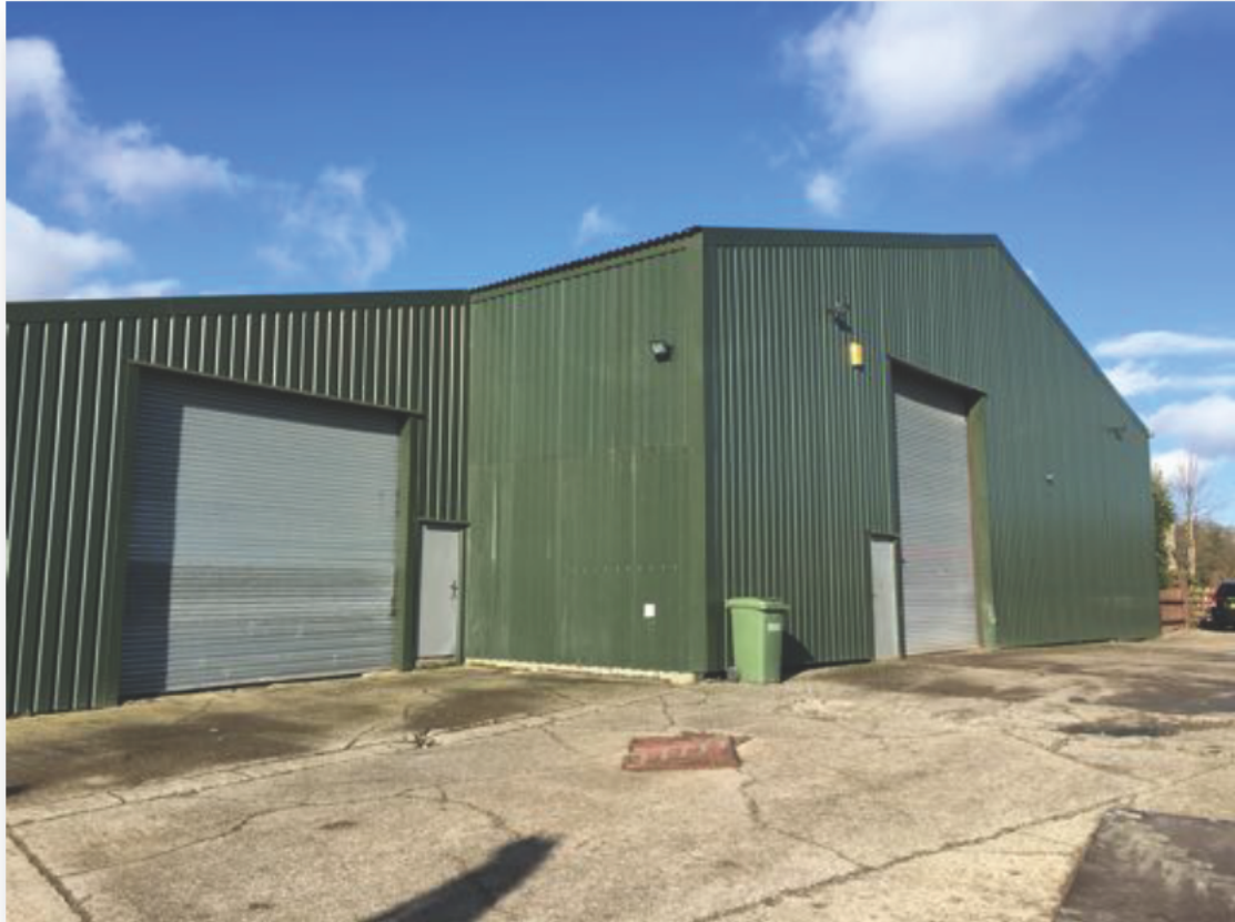
PHOTO 1: East Elevation of former portal-framed building (now removed by applicant)
