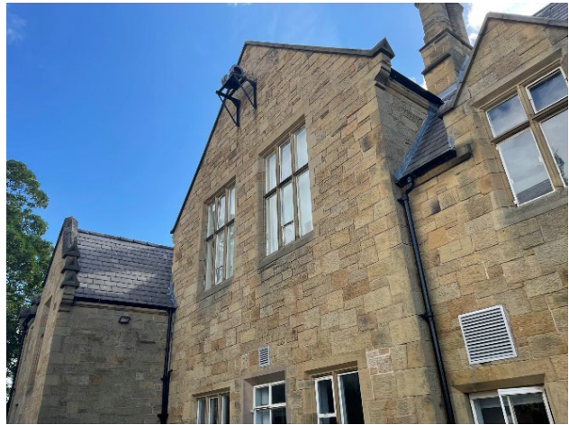
Photograph 4 – western aspect of building showing gable ends
