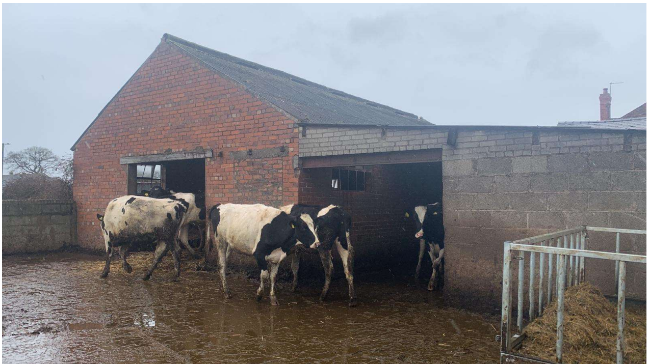
Existing poor quality livestock buildings at Ridleywood Farm
